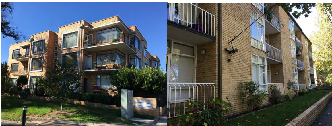
Figure 6.10–18 – Post-war flats – ‘Park View’, 126 Alma Road (left) and 22B Crimea Street (right)
