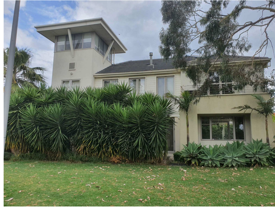
SUBJECT SITE VIEW FROM GARDEN CITY RESERVE
