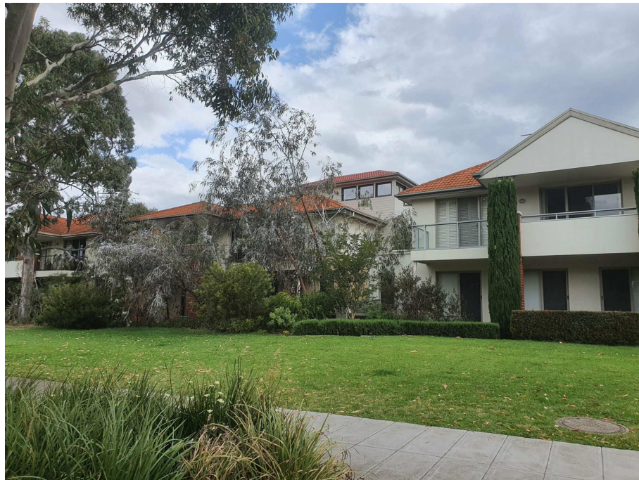
THREE STOREY HOUSE IN SAME SEGMENT FACING GARDEN CITY RESERVE
