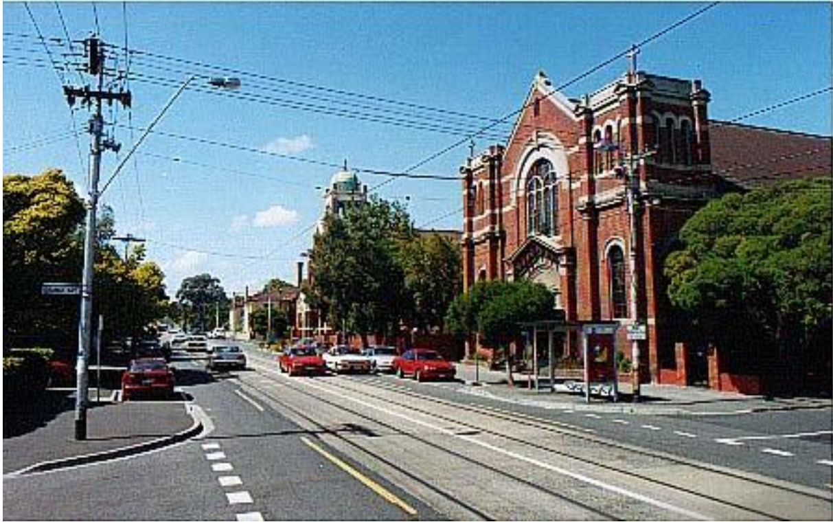
Figure 6.14-1 – Carlisle Street, looking east from the St. Colman’s Catholic Church and demonstrating their importance in the streetscape.
