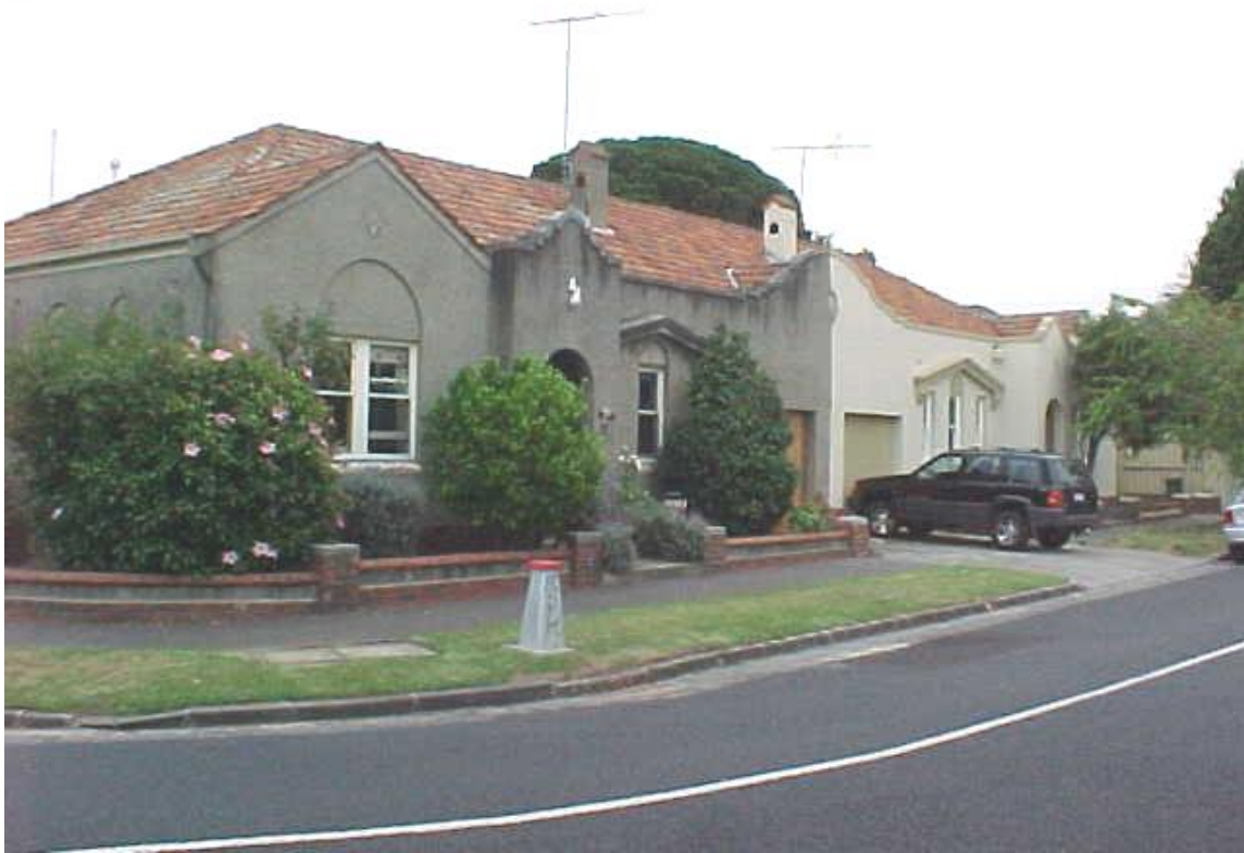
Figure 6.20-4 – II – IIa Hammerdale Avenue, East St Kilda (1932)
