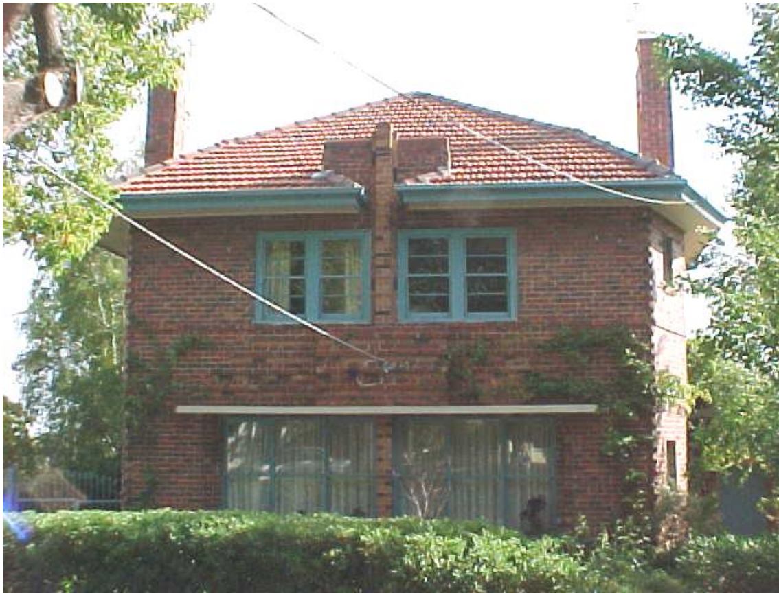
Figure 6.21-4 – Duplex, 2 – 3 Holroyd Court (1938)
