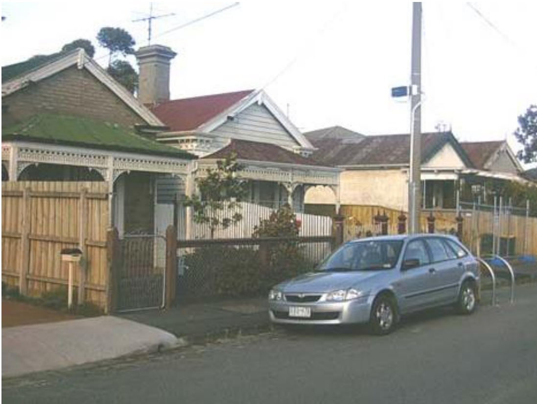
Figure 6.30-4 – Row of single-fronted gable-ended timber cottages at 10-18 Gibbs Street (note development site at No 14)
