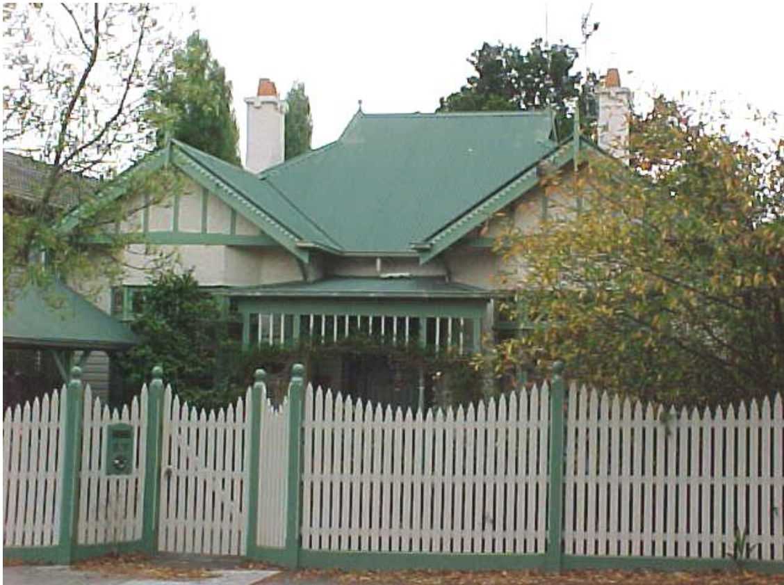
Figure 6.22-5 – Weatherboard house at No. 27 Kalyrna Grove, East St Kilda
