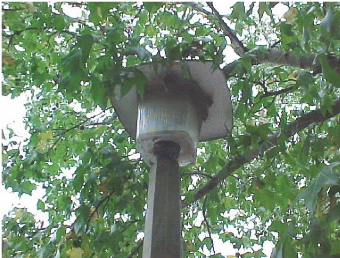
Figure 6.23-5 – Detail of 1920s concrete lamp
