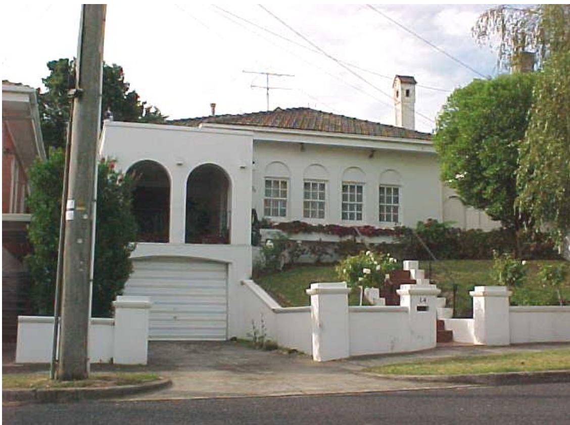
Figure 6.23-3 – House at 14 Mooltan Avenue (c.1928)
