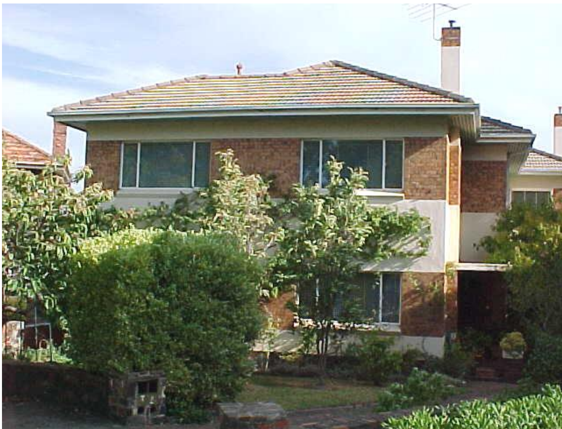
Figure 6.21-5 – Duplex, 4 – 5 Holroyd Court (1939)
