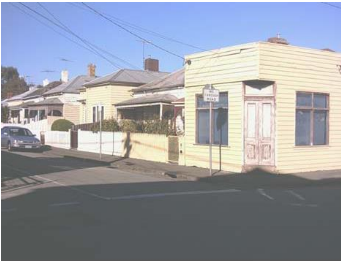
Figure 6.30–6 – Hip-roofed timber cottages in Marlborough Street, with weatherboard corner shop (c.1890) at No 31
