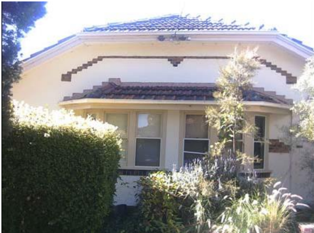
Figure 6.29-2 – Unique gambrel-roofed house at 4-6 McCrae Street, note: canted bay window across both dwellings
