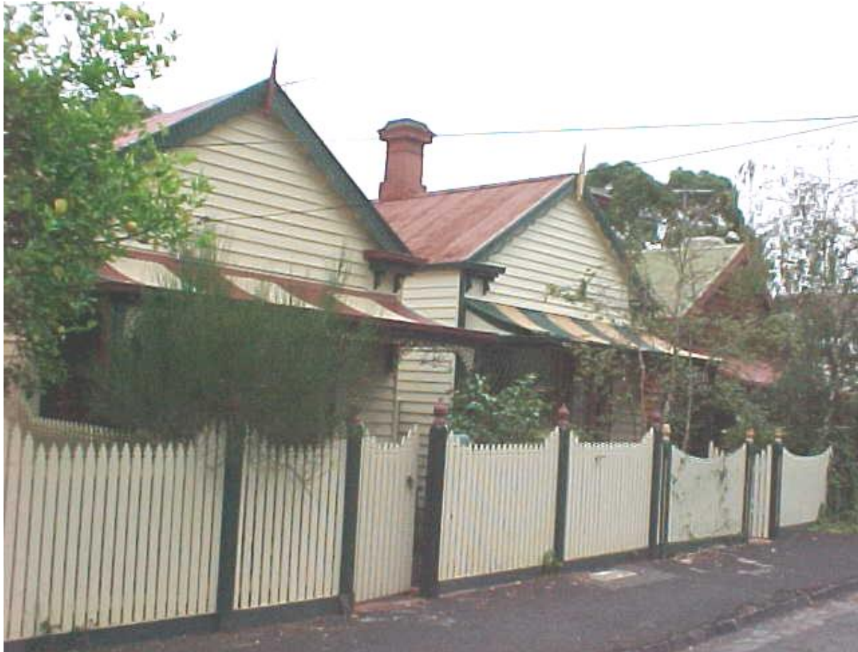
Figure 6.18-2 – Chusan Street, East St Kilda - looking north
