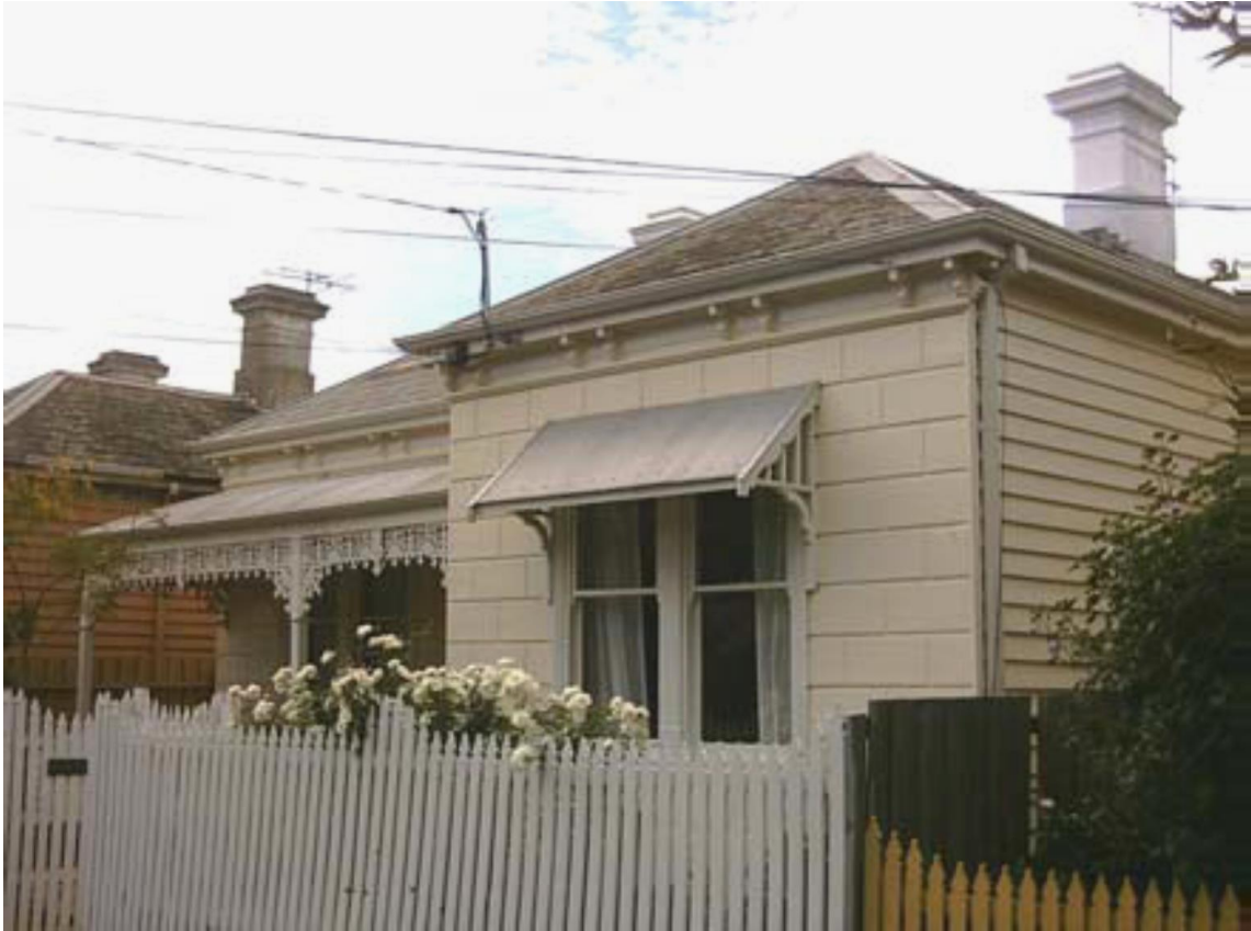
Figure 6.28–5 – Typical double-fronted timber villa, one of several in a row in Moore Street
