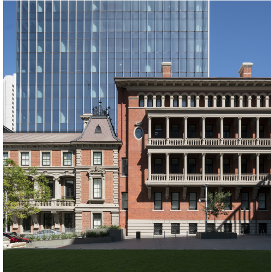
KERRY HILL ARCHITECTS - COMO, THE TREASURY, PERTH
