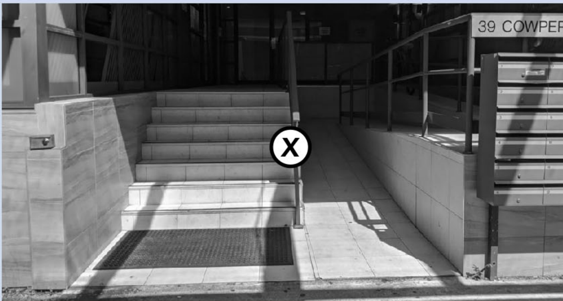
Figure 45: A long ramp into the building can create a dark entrapment space.
