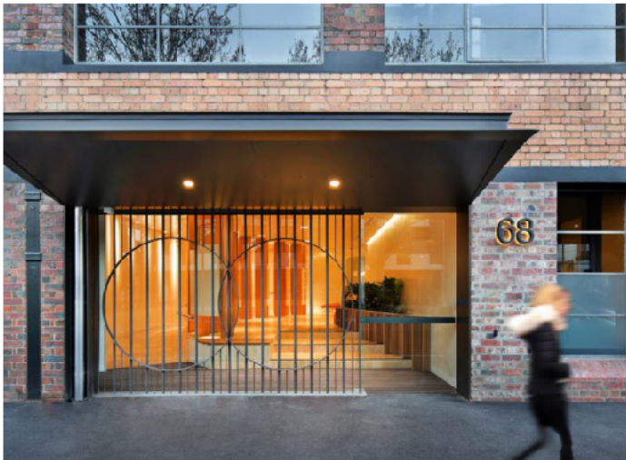
Figure 49: This apartment building integrates an internal ramp and stairs into the entry lobby design. A large opening to the street and lighting provides visibility through the building.
