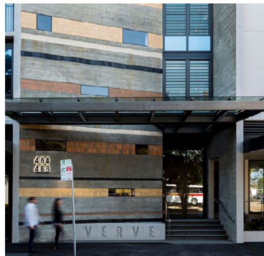
Figure 65: Concrete plinth with integrated building signage and a raised planter bed provide a flood resilient base to the elevated entrance to this apartment building.
