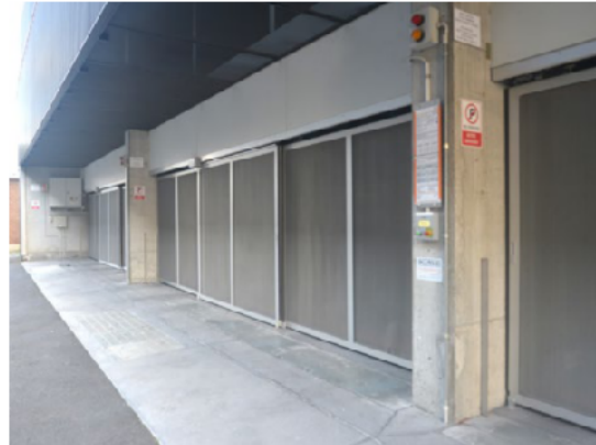
Figure 69: Self-actuating vertical-rise flood barriers protect these garages with car stackers in a South Melbourne laneway.
