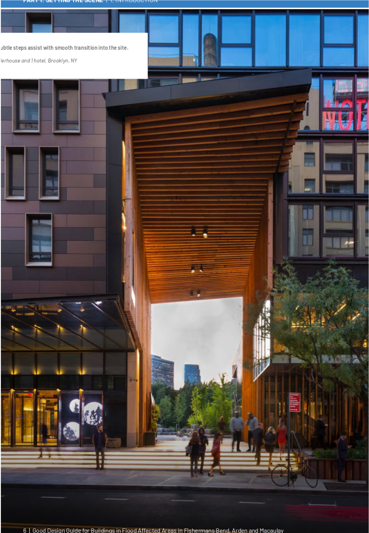
6 | Good Design Guide for Buildings in Flood Affected Areas in Fishermans Bend, Arden and Macaulay
