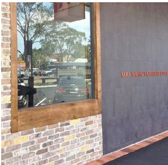
Figure 64: Specialist flood-resilient window and glazing assembly to restaurant window.
