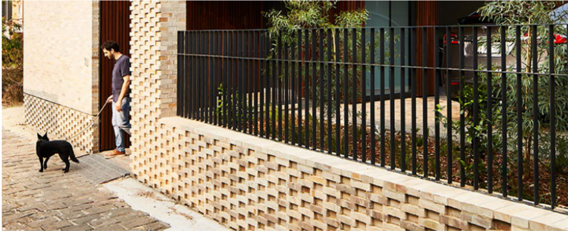
Figure 63: Finely detailed brickwork in front of a waterproof substrate provides a flood resilient base to the canal frontage of these new townhouses. Windows, doors and balconies are all elevated above the flood level.
