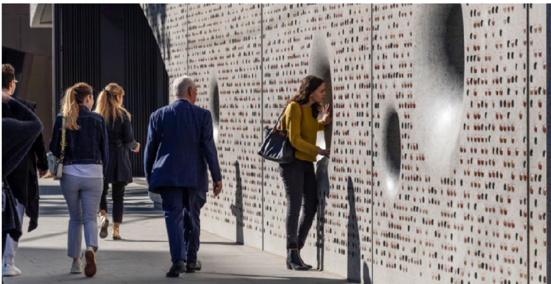
Figure 10: Playful, human-scaled windows invite engagement with the passing public. The concrete base of the wall provides protection from floodwaters.
