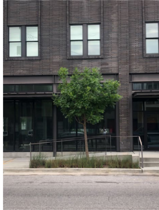
Figure 15: Raised footpath along a section of the street allows for accessible transition between two levels.
