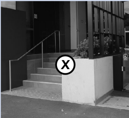
Figure 34: The presentation and legibility of the main entry to the building is compromised because it is recessed from the street. An external platform lift is not a preferred outcome
