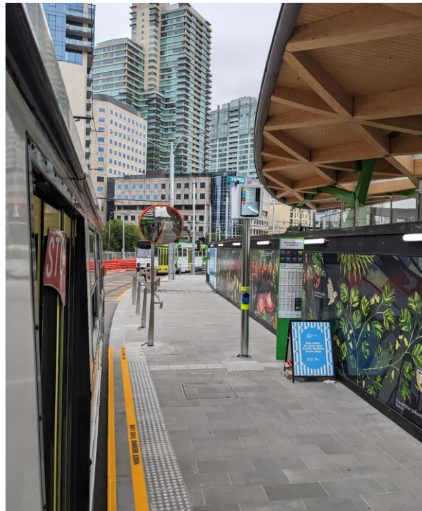
Anzac Station central platform (Northbound)
