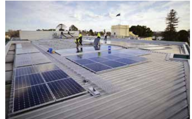
Solar panel installation at Port Melbourne Town Hall.
