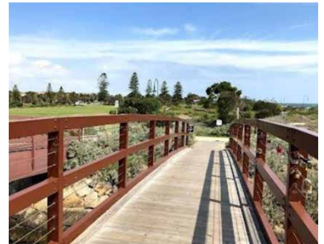
Moran Reserve Bridge, Elwood.
