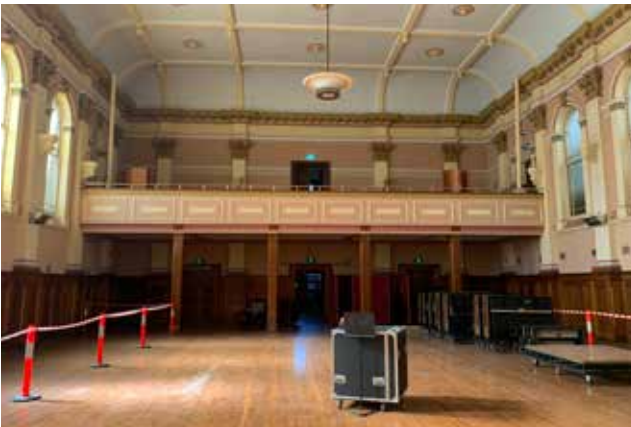
Site investigations for the South Melbourne Town Hall's renewal and upgrade.
