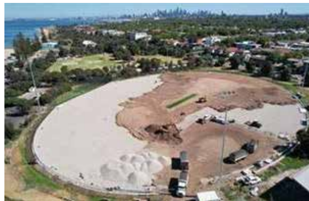
The oval redevelopment includes the levelling of the new ground profile.
