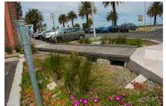
Raingardens help improve water quality by trapping litter and filtering invisible pollutants.
