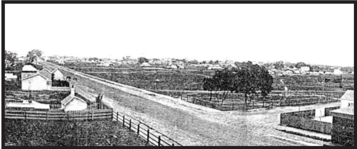
Figure 6.11-5 – Carlisle Street, looking west from the railway bridge c.1862.
