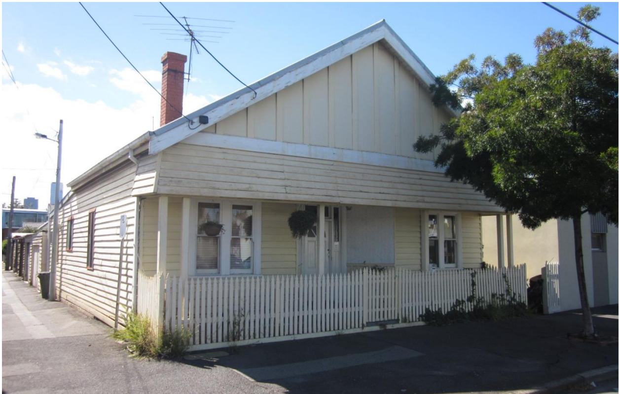
Figure 6.3–10 – Atypical early 1920s timber bungalow at 234 Bridge Street.
