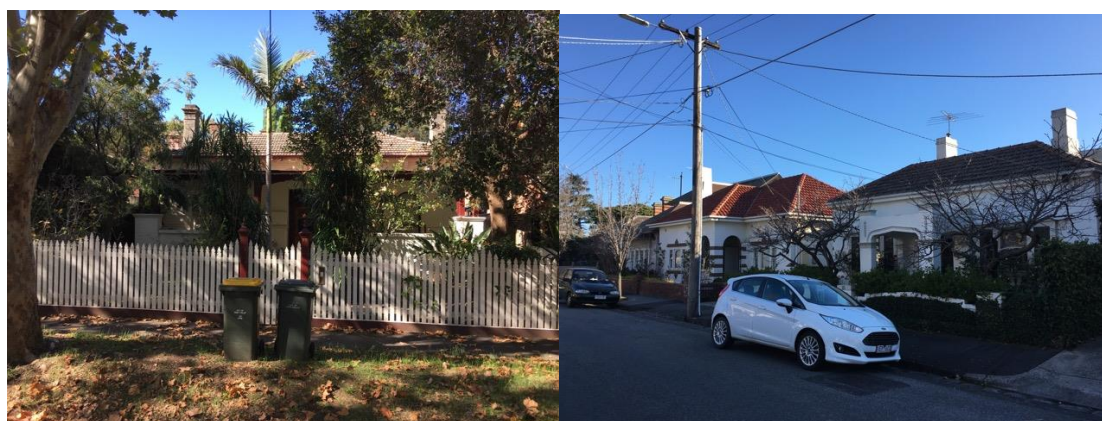
Figure 6.10–13 – Victorian villas with interwar makeovers – 28 Crimea Street (left) and 10 & 12 Shirley Grove (right)
