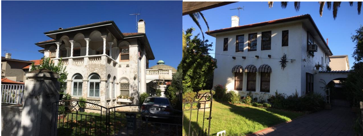
Figure 6.10–17 – Spanish Mission style – 11A Charnwood Road (left) and 151 Alma Road (right)
