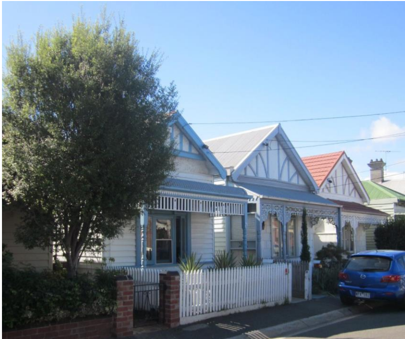
Figure 6.3–9 – 25-29 Albert Street, three of a row of eight Federation-era cottages, set to the south end of the street.
