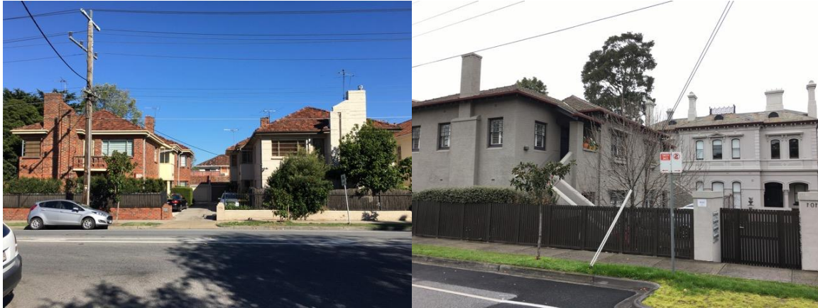
Figure 6.10–16 – Moderne flats at 119A & 121 Alma Road (left), interwar bungalow flats and Victorian mansion at ‘Sandhurst Court’ (right)
