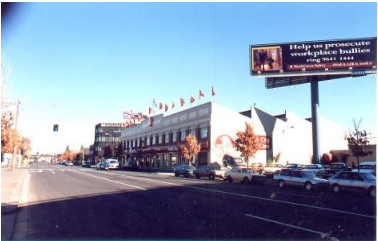
Figure 6.8–6 – Former General Motors Corporation headquarters, City Road, looking towards the railway overbridge.
