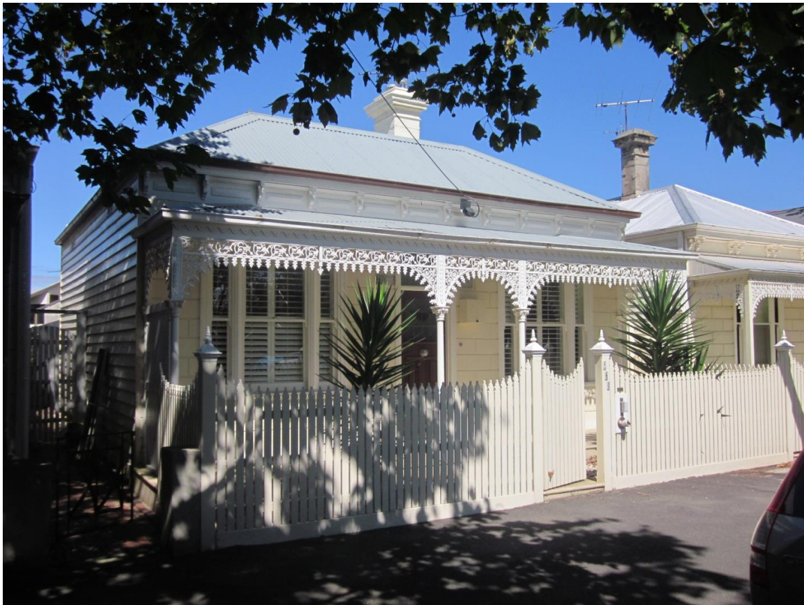
Figure 6.3–6 – Late Victorian block-fronted timber villas in Clark Street – a street with ‘Avenue’ characteristics.
