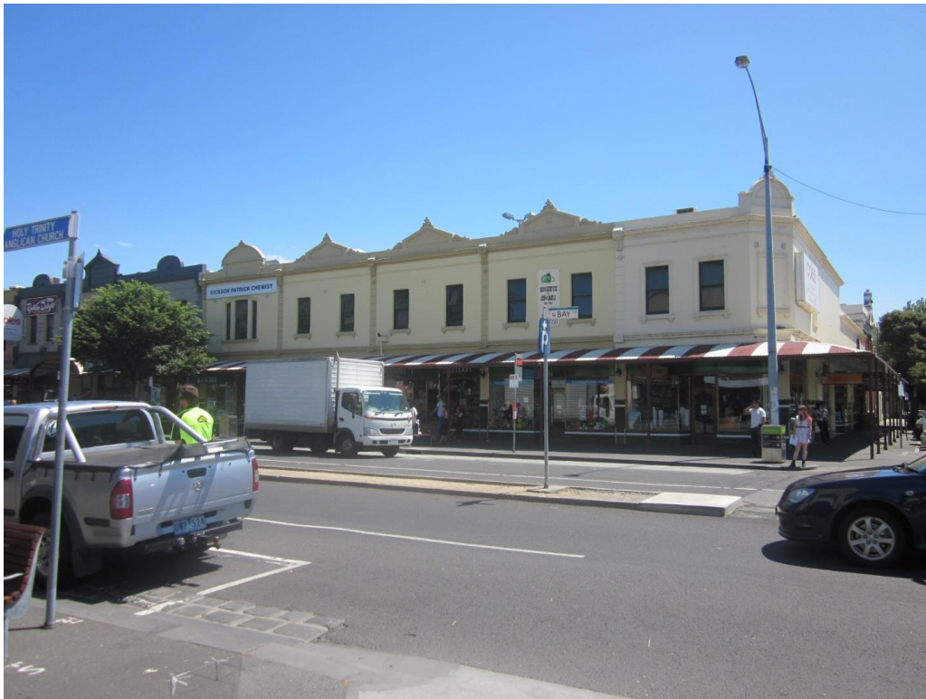
Figure 6.5-2 – The market buildings at 191-219 Bay Street
