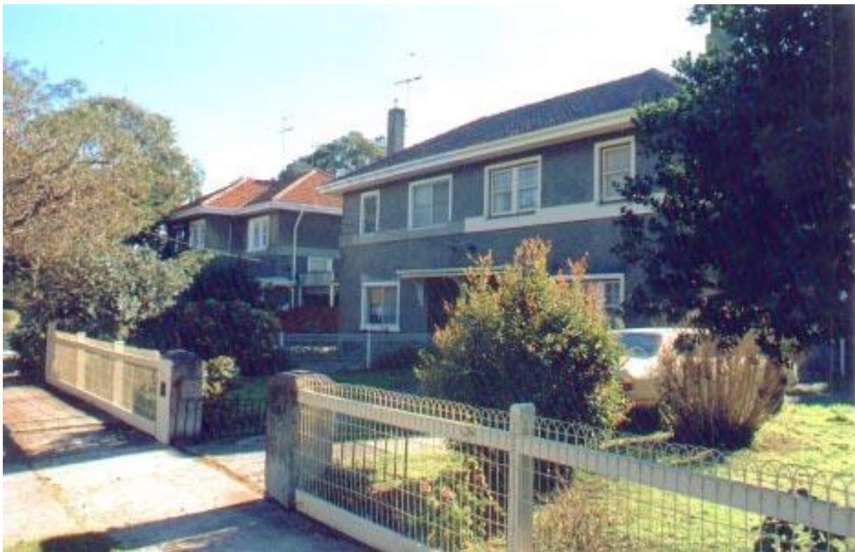
Figure 6.7-4 – Unpainted rough cast duplex units in Crighton Avenue, complete with crimped wire front fences.
