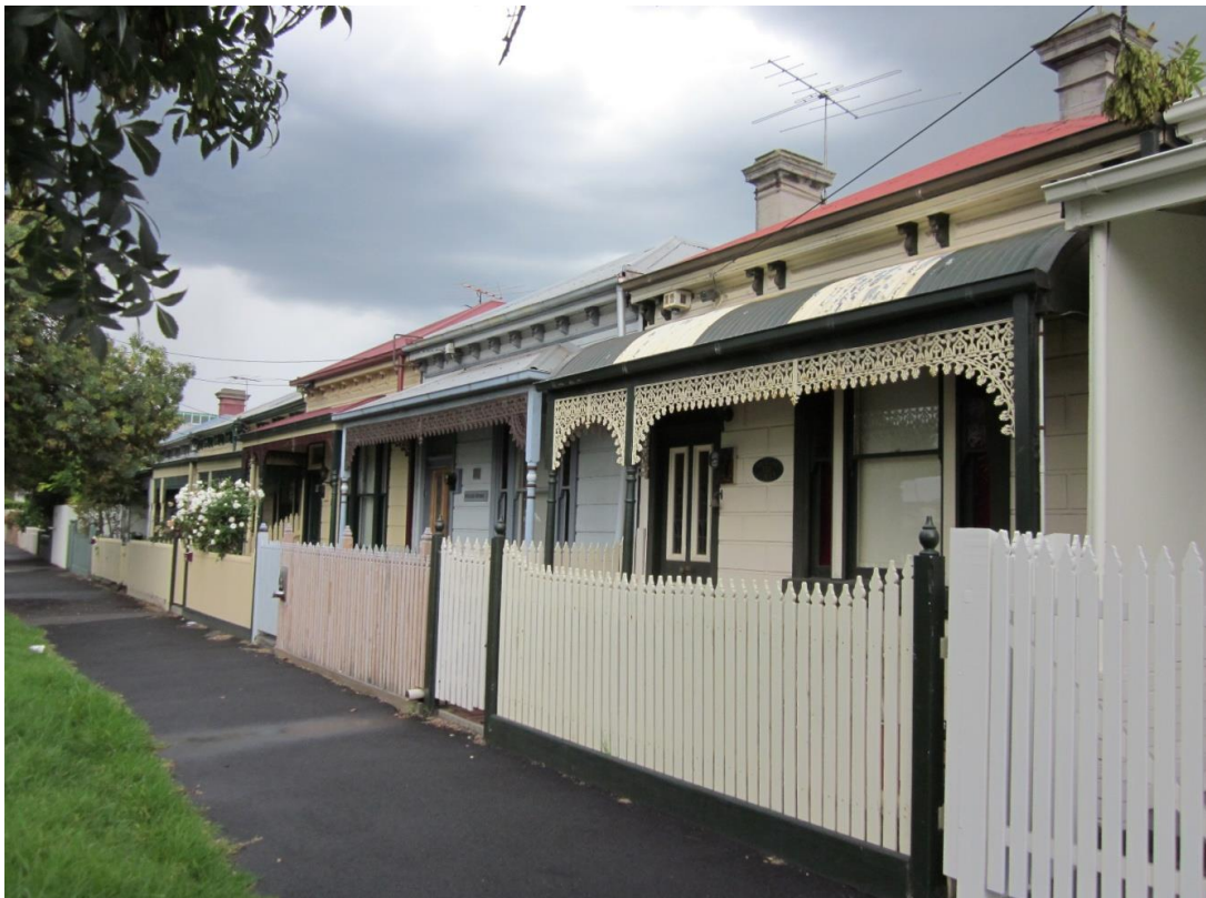
Figure 6.4–3 – Single-fronted dwellings in Pickles Street.
