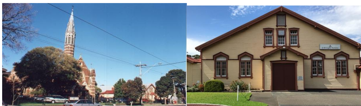
Figure 6.10–8 – St. George's Uniting (former Presbyterian) church of 1877-80 and the former St. Kilda Orderly Room dominate the Chapel Street hill
