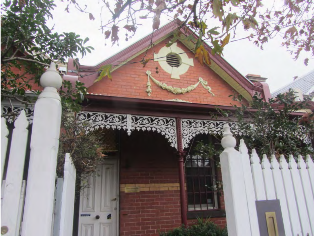
Figure 2. Showing decorative detailing common to 110-112 Barkly Street and 2-6 Blanche Street (oculi and swagged garlands on gable end, verandah posts and cast iron frieze, cream brick banding).
