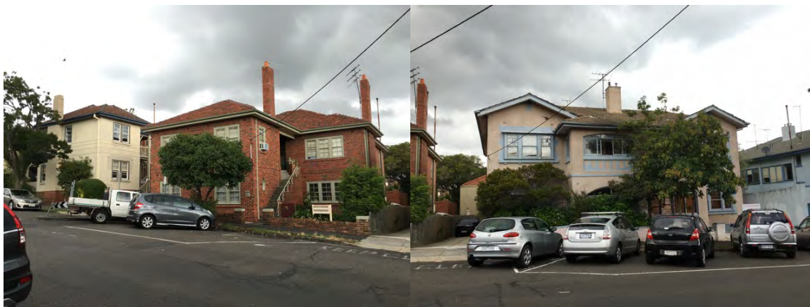
Figure 1 At left are 39 Mitford Street (pale rendered building) and 41A Dickens Street (red brick), within HO7, while at right is no.41 Dickens Street, outside HO7
