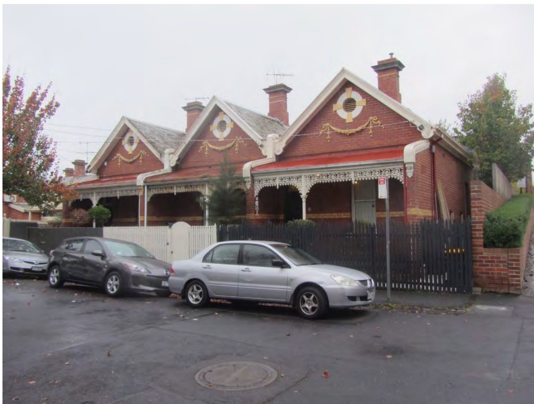
Figure 4. 2-6 Blanche Street showing the identical form and detailing of this conjoined group of three houses, and the high degree of intactness.
