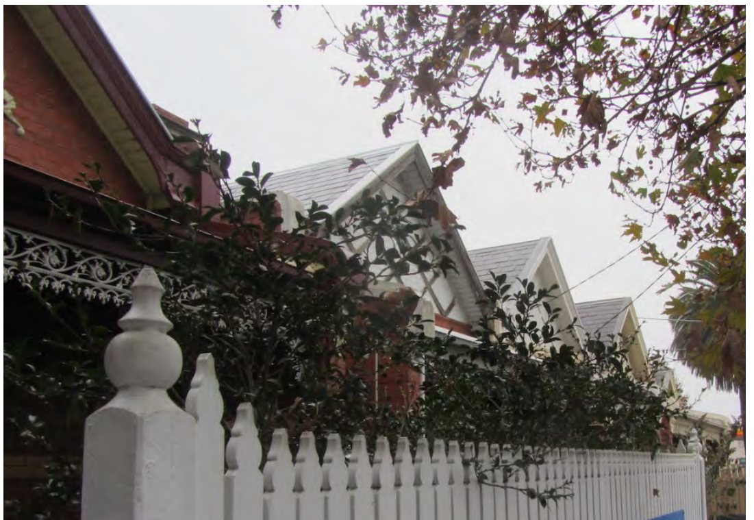
Figure 6. 114-118 Barkly Street, showing slate roofs to all, and alternate gable end decoration on 114-116 Barkly Street.
