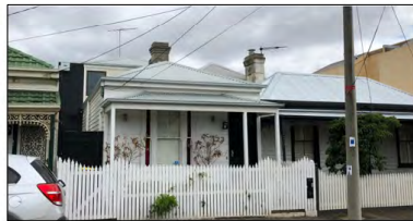
127 + 123 ALBERT STREET OPPOSITE THE SUBJECT SITE, OF SIMILAR HERITAGE CHARACTER WITH REAR TWO-STORY EXTENSION.
