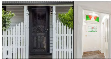
EX.003 REINSTATED ORIGINAL VICTORIAN STYLE PANELLED DOOR WITH TOPLIGHT FINISH: PAINTED AS PER ORIGINAL LOCATION: FRONT FACADE
