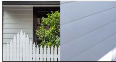
EX.002 WEATHERBOARD CLADDING (SQUARE-EDGED) FINISH: PAINTED AS PER ORIGINAL LOCATION: FRONT FACADE WALLS + SIDE FACADE WALLS AT EXISTING PORTION OF HOUSE
