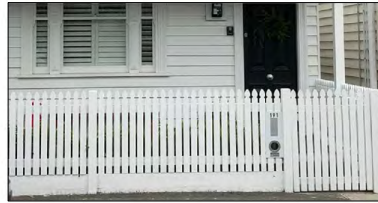
A.300 TIMBER PICKET FENCE FINISH: PAINTED AS PER ORIGINAL LOCATION: FRONT FENCE
