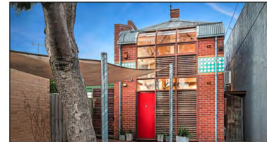
8 CLAY STREET. LOCATED AT THE REAR OF THE SUBJECT SITE, AN ECLECTIC BRICK + TILED TWO-STORY DWELLING WHICH CONTRIBUTES TO THE DIVERSE STREETSCAPE + NEIGHBOURHOOD. ITS NORTHEAST PARAPET WALL DEFINES THE REAR BOUNDARY OF THE SUBJECT SITE.
