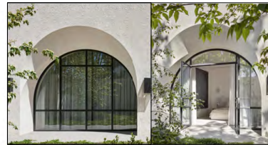
A.502 STEEL DOORS FINISH: BLACK STEEL FRAMES, CLEAR GLASS LOCATION: REAR FACADE AT GROUND FLOOR
