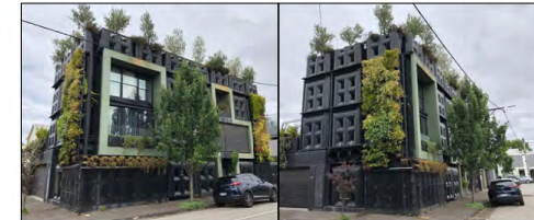
CORNER OF UNION ST + ALFRED ST. THE 'PORT MELBOURNE URBAN GREEN HOUSE' IS A UNIQUE DWELLING CONSTRUCTED FROM RAIN WATER TANKS AND LOCATED WITHIN CLOSE PROXIMITY TO THE SUBJECT SITE.
