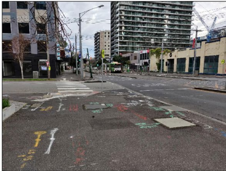
Photo 3: Park Street and Palmerston Crescent intersection – facing west
