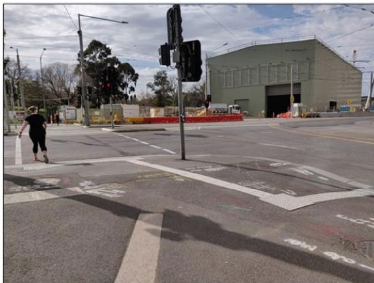
Photo 10: Park Street at St Kilda Road intersection – facing east
