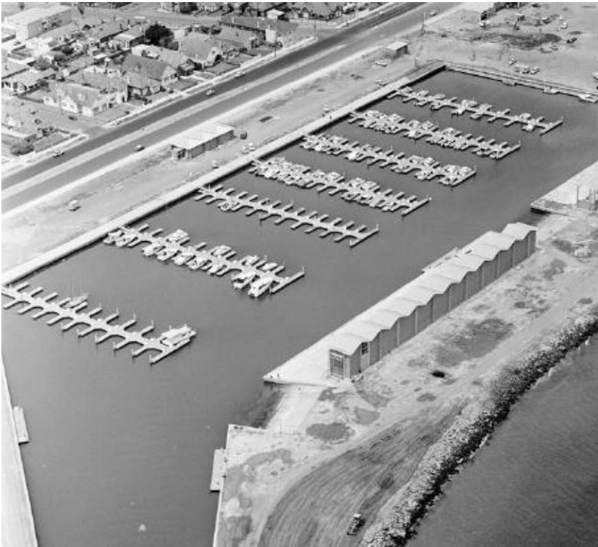
Figure 1 - Marina site circa early 1969, showing moorings, one completed dry boat storage building (with another under construction). Note, on far side of harbour, the amenities block, substation and petrol station.
