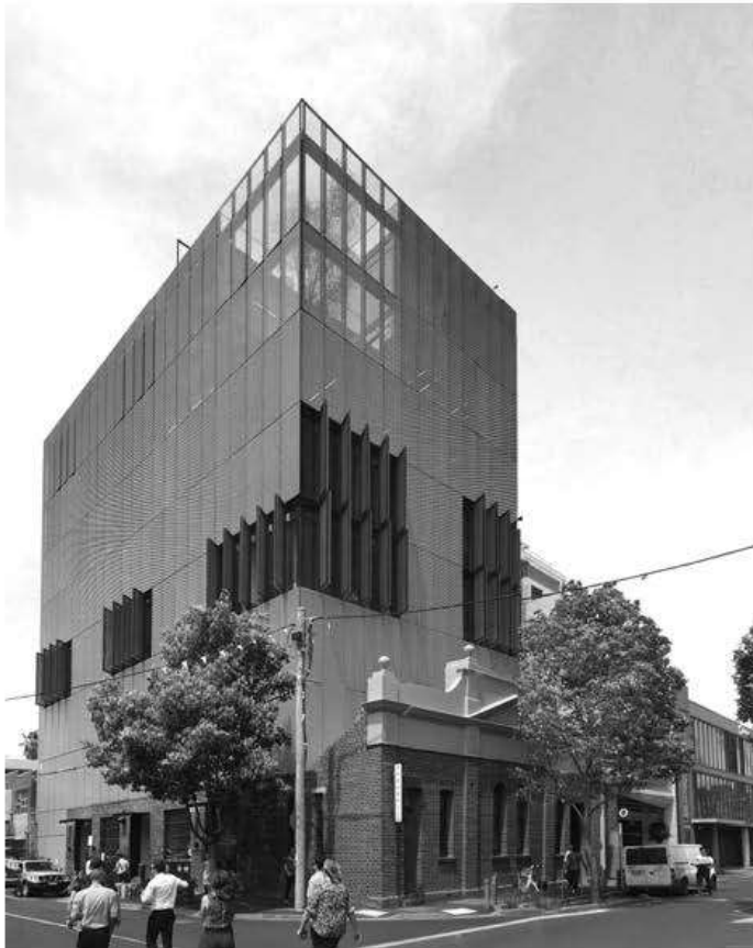
Photo 12. Lightweight material and simple details used for an office addition above a Federation era factory of local significance in Cremorne Street, Richmond. While the front setback of this addition is less than recommended by the guide lines, the visual impact is mitigated using lightweight materials and simple form and detailing, which ensures the heritage building remains legible.
