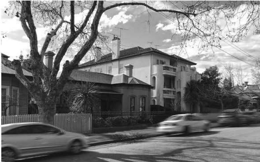
Photo 8. An example of a diverse streetscape consisting of various Contributory places of different eras
