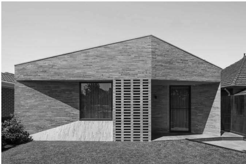
Photo 16. Ground Floor Facade of Bayside House, Adam Kane Architect
