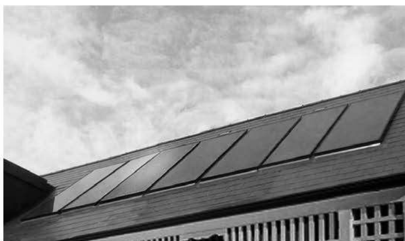
Photo 22. An example of frameless solar panels on a slate roofed building
