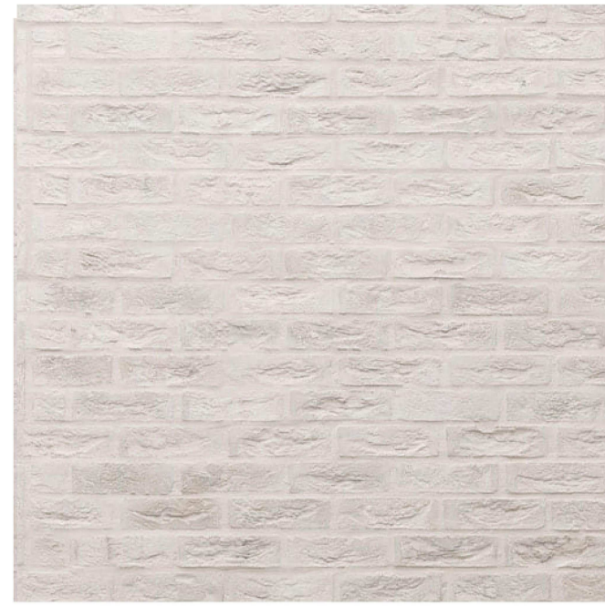
CODE: BR1 MATERIAL: BRICK WORK FINISH: BAGGED TEXTURE FINISH LOCATION: EXTERNAL WALLS AS INDICATED
