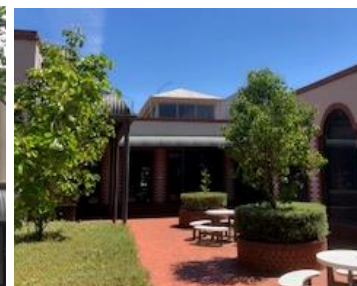
Partial rear view
