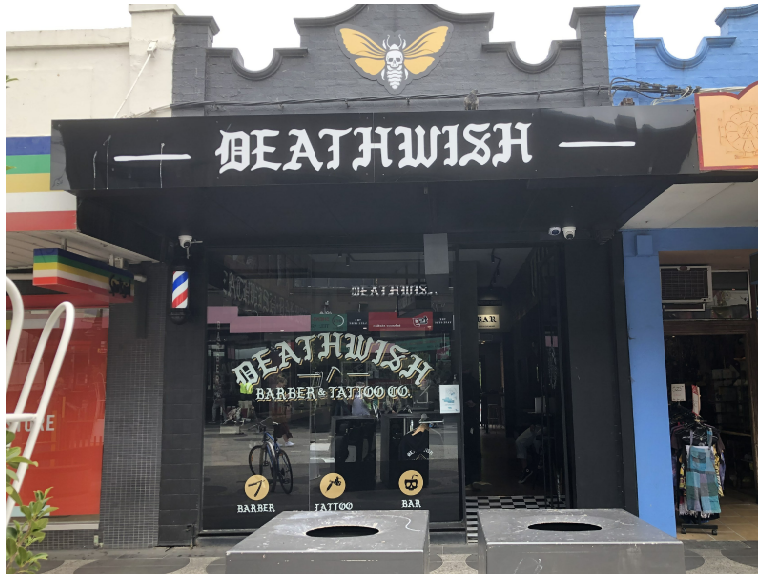
Existing Street Facade
