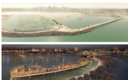
St Kilda Pier Redevelopment
