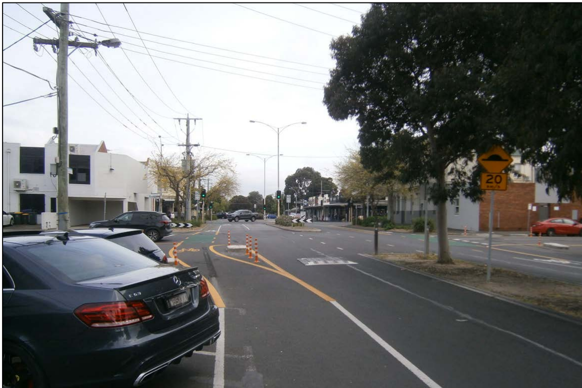
Figure 12: Realignment of Bridge St Westbound Bike Lane on Approach to Lyons St
