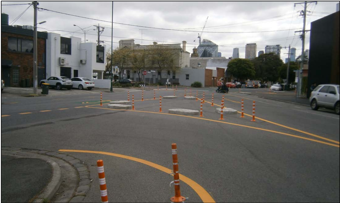
Figure 10: Splitter Island Comprising Concrete Blocks and Bollards on Esplanade West Approach to Lyons St
