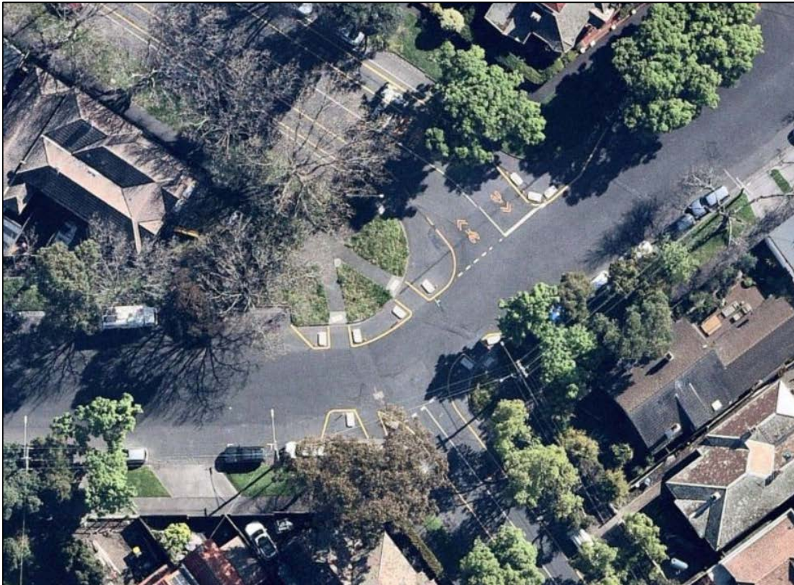
Figure 8: Concrete blocks at Deakin St/Loch St and Deakin St/York St Intersections
