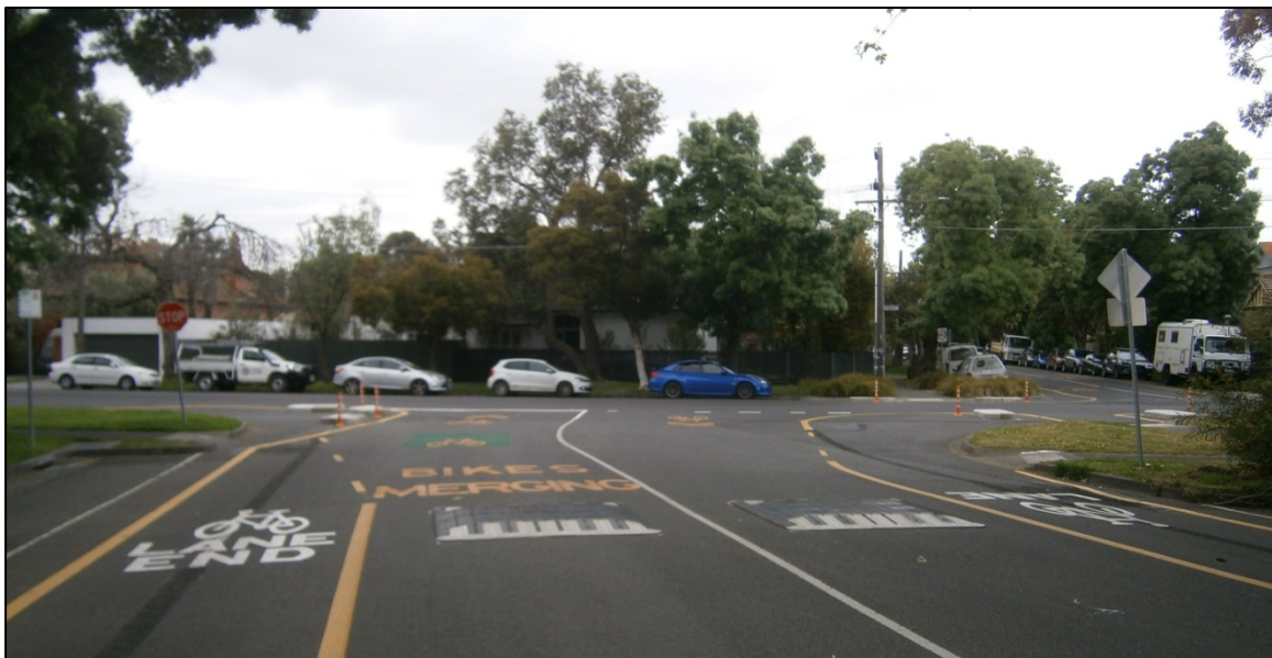
Figure 6: York St Approach to Deakin St Looking South
