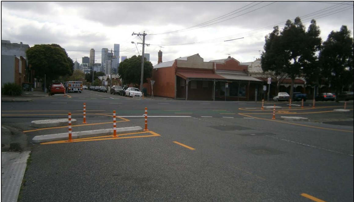
Figure 11: Narrowing of Lyons St South Approach to Bridge St
