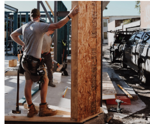
Construction site of townhouse development. Photography by Sunlyt Studios
