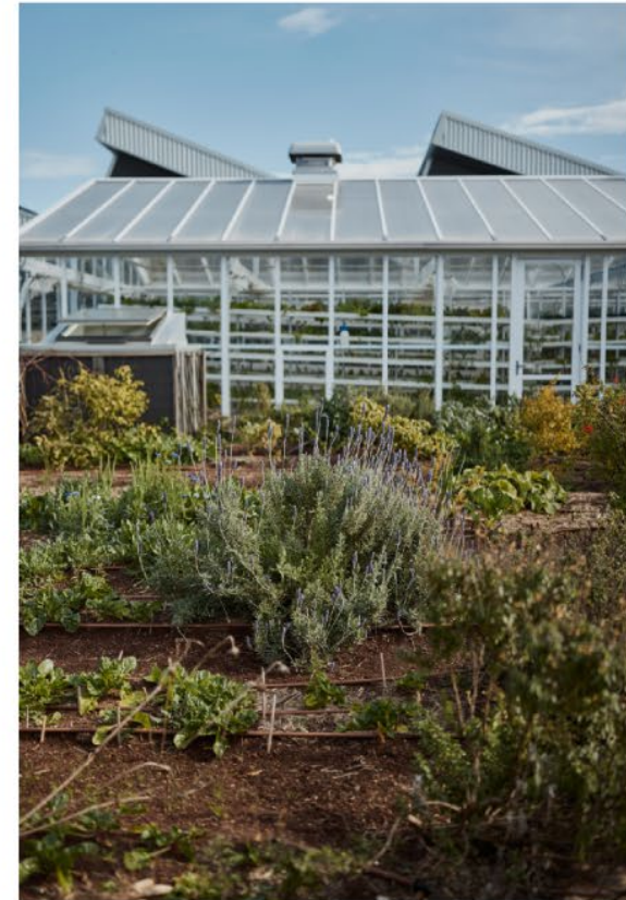
Rooftop garden and solar photovoltaic panels at Burwood Brickworks. Photography by Kim Landy
