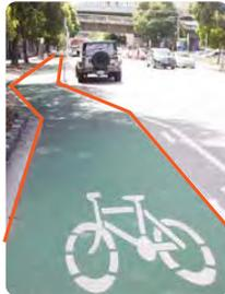
**Protected bike lanes** have been recently constructed on Moray Street creating a high quality buffer to protect cyclists from parking cars, 'car-dooring' and vehicles in motion. DoT have more planned for St Kilda Road as they have proven popular with cyclists.
