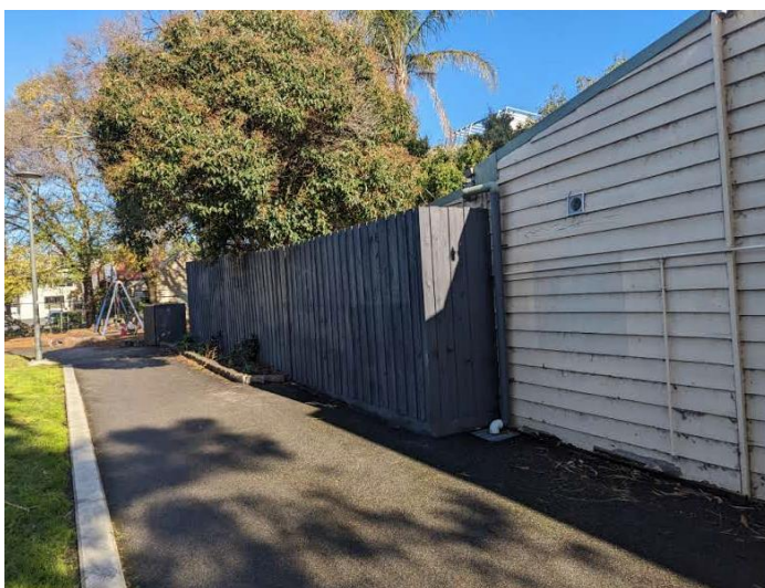
Figure 3 – Subject site 43 Pakington Street St Kilda (Site visit image taken by M Nuciforo 19-6-2023)
