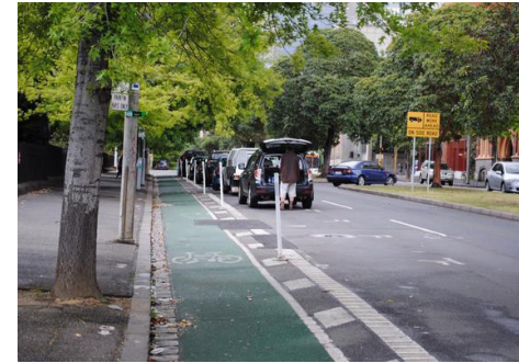
Example of temporary road arrangement at Albert Street, East Melbourne. Photos: Lorenza Casini
