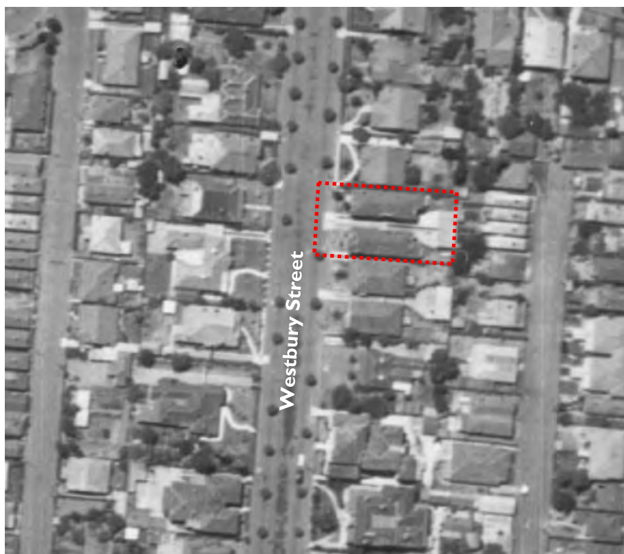
Figure 4 - Aerial photograph dated 1945. Subject site is outlined. (Source: Landata, Proj No 5, Melbourne and Metropolitan Area Project, Run 17E, Frame 58013)
