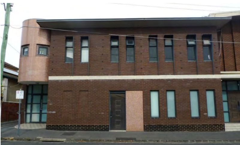
North Elevation, 1996 addition
