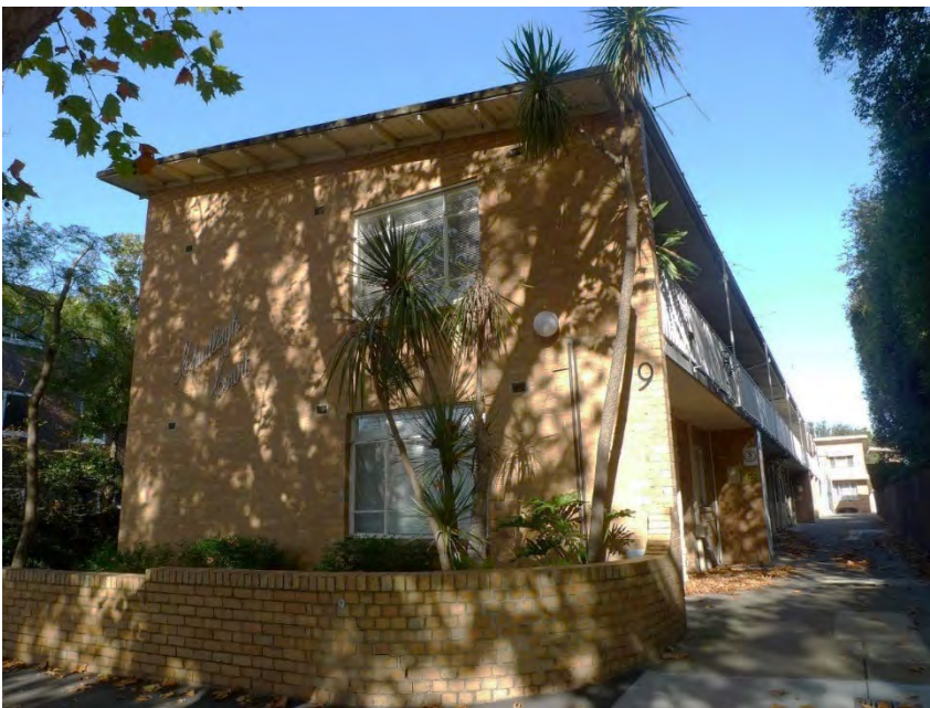
Building from the west side
