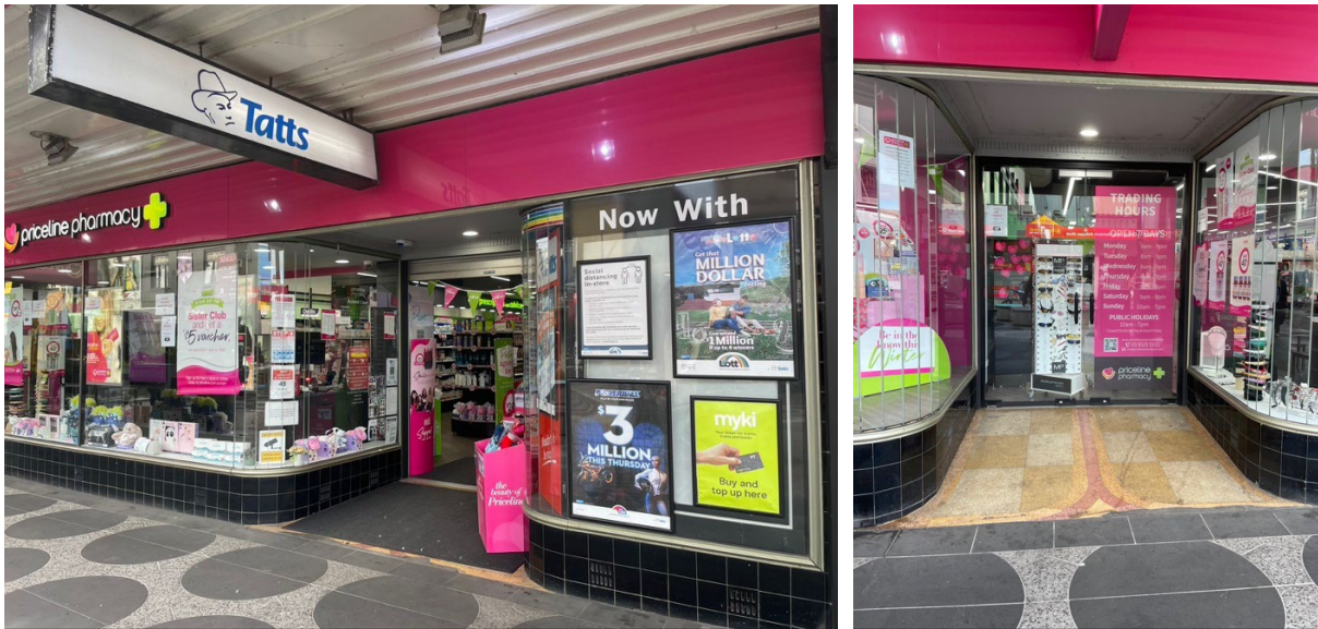
Original shopfronts to Acland, showing (at right) terrazzo floor to the ingos (covered by mat in left image)
