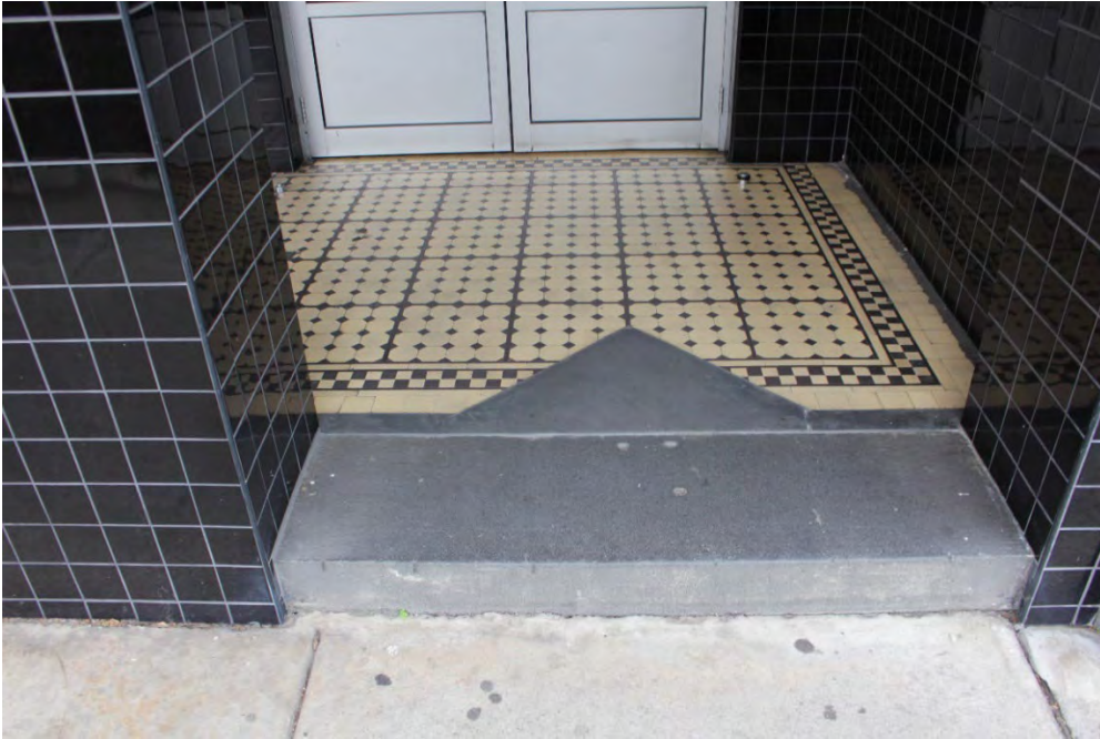
Basalt threshold and original cream and black tiling to the deck
