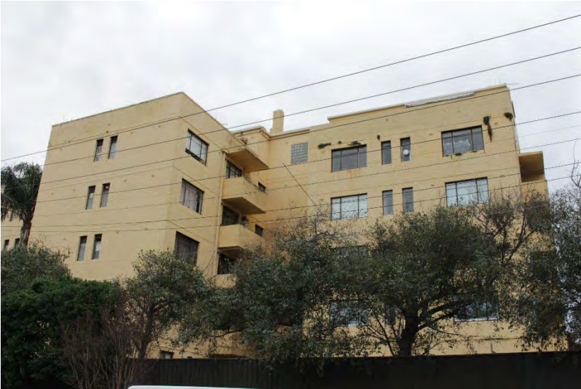
South Elevation – east end (Argyle Street)
