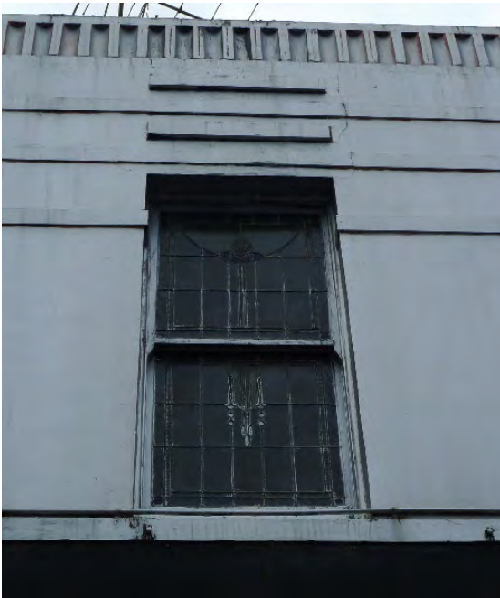
South side, window with decorative leadlight glazing
