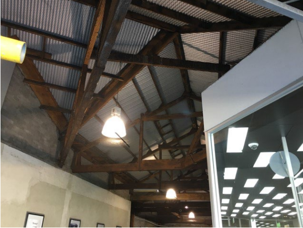
Internal roof trusses within former car shed
