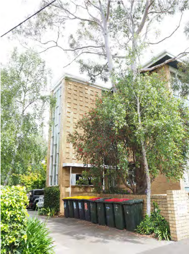
Circulation tower with staggered glazing bars
