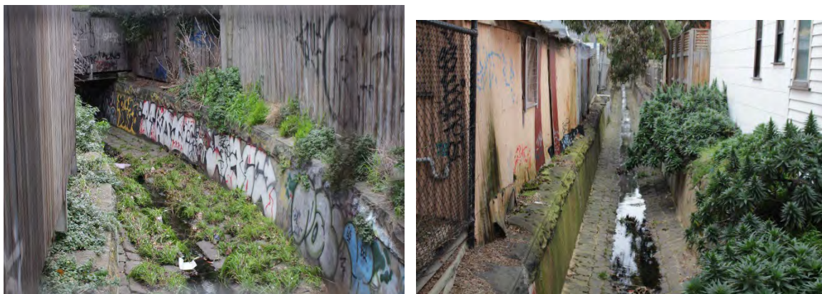
Figures 18 & 19 – section of early bluestone drain west of Lynott Street (left) and east of Lynott Street (right)
