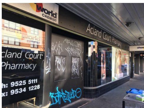
Barkly Street elevation and shopfront
