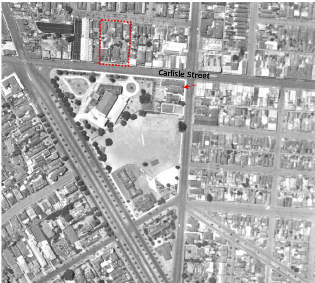
Figure 21 - 1945 aerial photograph, west end, houses where library now stands are highlighted, and Methodist hall (Source: Landata, Proj No 5, Melbourne and Metropolitan Area Project, Run 17E, Frame 58012)
