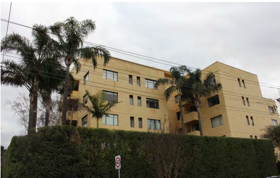
South Elevation – west end (Argyle Street)
