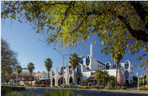
The Victorian Pride Centre was commended for its sustainable design as part of Council's recent Design and Development Awards
