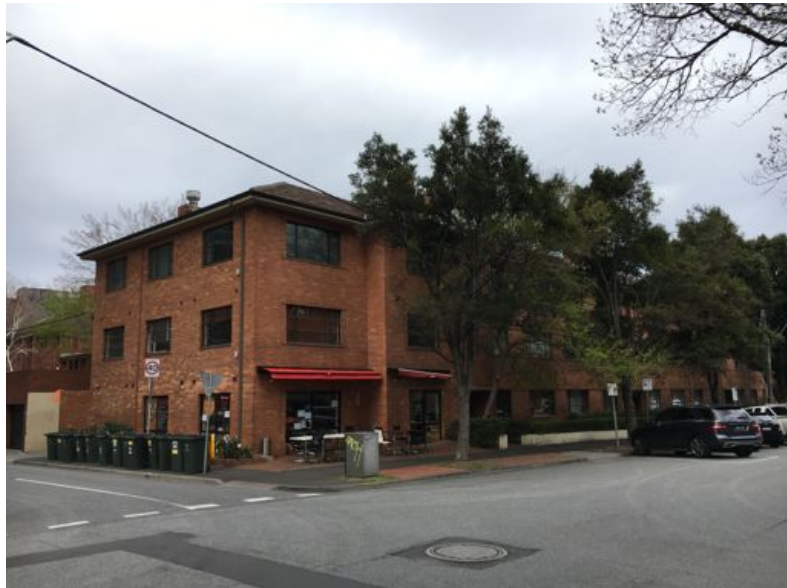
The rear of Glen Eagles and its ground floor shop, viewed from the corner of Beatrice Street and Queens Lane.
