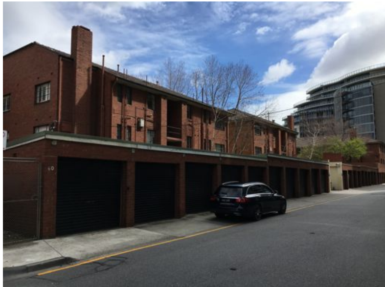
The rear of Kinfauns and Kinross, viewed from Queens Lane. Visible in the foreground are the 23 single-car brick garages of the complex. The rear of Glen Eagles is partially visible at right.
