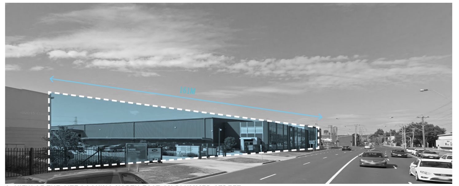
2. VIEW OF THE SITE LOOKING NORTH EAST ON PLUMMER STREET
