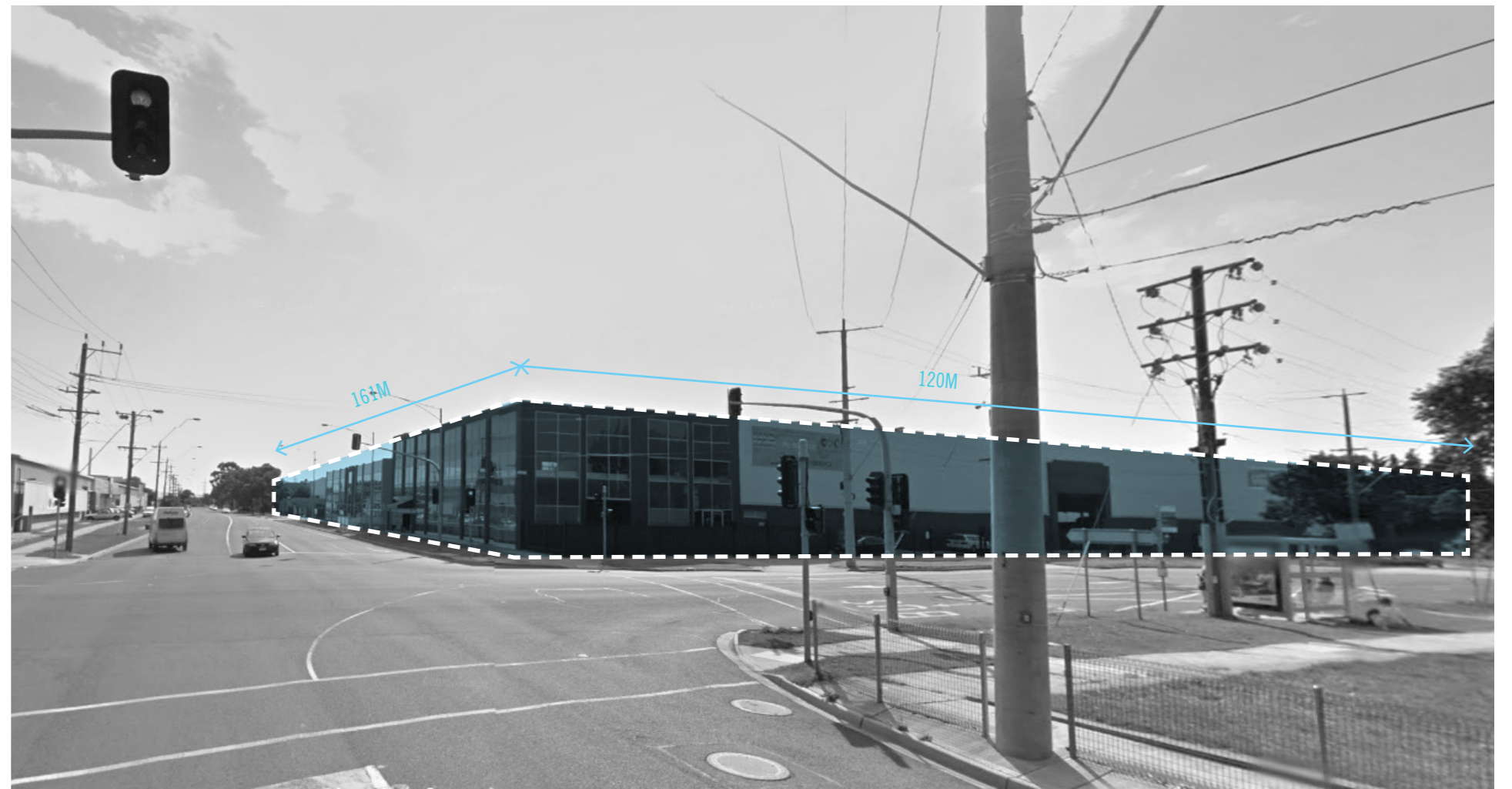
VIEW OF THE SITE LOOKING SOUTH WEST FROM THE CORNER OF PLUMMER ST & SALMON ST
