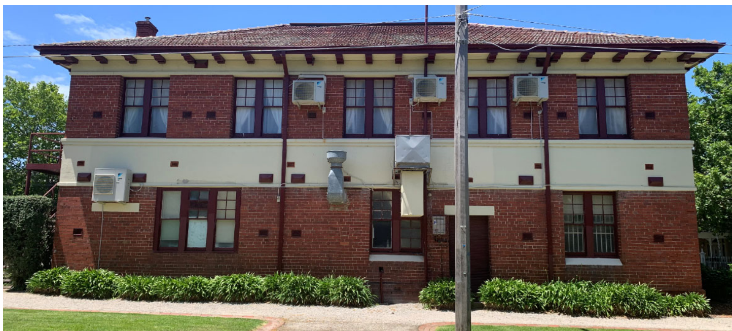
Image above: photo of rear (western side) of the subject building. Note the bowed roof, suggesting structural distress, and the unsympathetic additions of air-conditioning units and venting.
