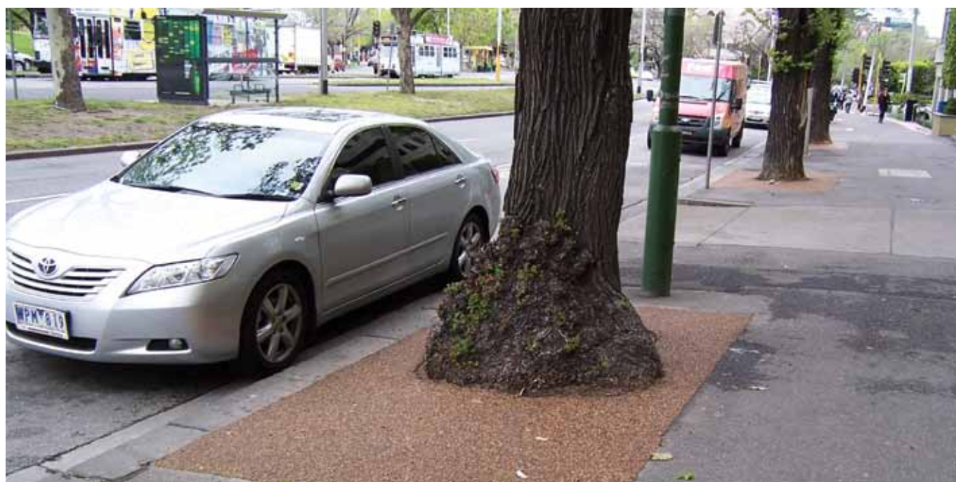
Porous pavement on St Kilda Road allows water through and protects the roots of the Elm tree
