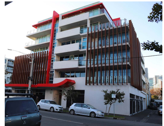
Balconies siding onto Nott Street setback 0.0m from the boundary at 203 Rouse Street
