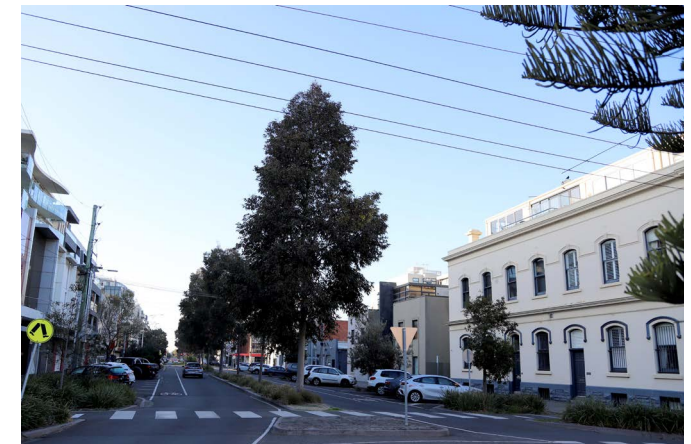
Rouse Street with bike lanes, parking and pedestrian crossing, looking north-east
