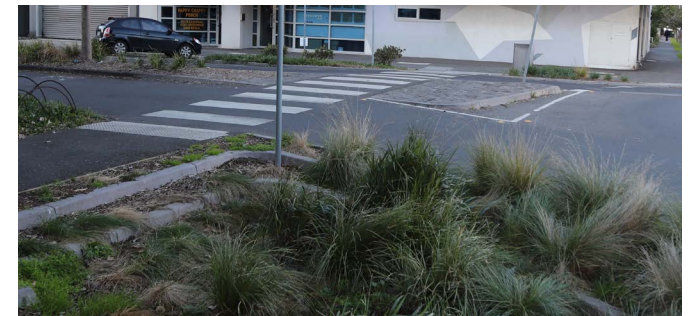
Raised pedestrian crossing, quality materials and enlarged WSUD verges create a pleasant environment along Rouse Street
