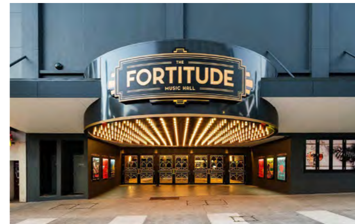
Fig. 1.5 Fortitude Music Hall, Brisbane, QLD Source: Concrete Playground
