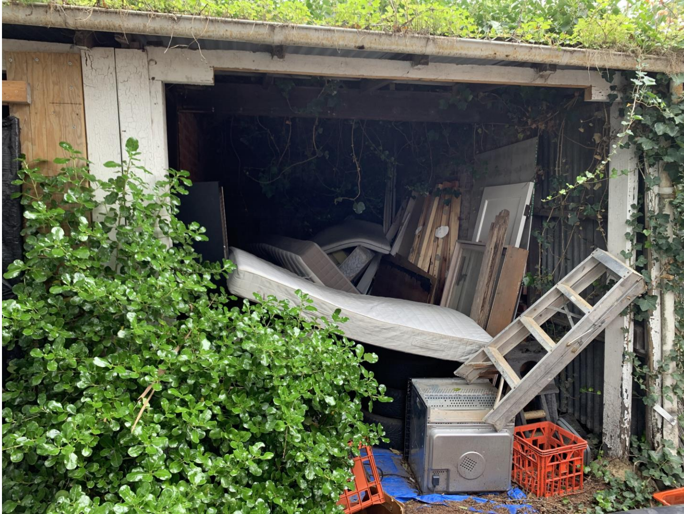
Image 8: Garages to the rear of the building. Source: M. Cooksley, 2020
