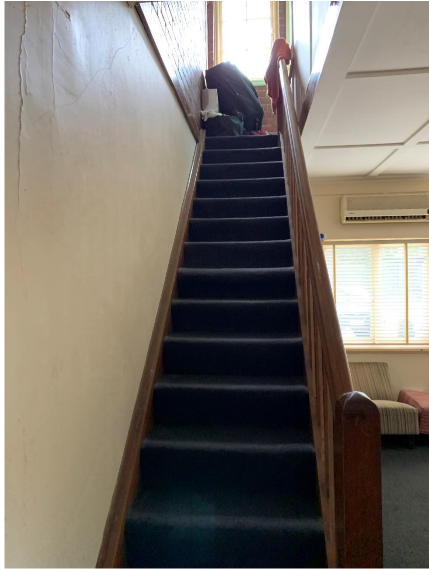
Image 6: Staircase from ground floor to first floor. Source: M. Cooksley 2020
