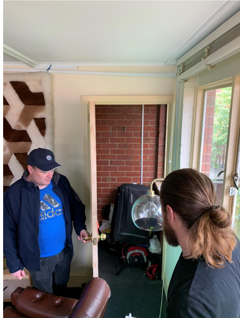
Image 7: Door at top of staircase. Source: M. Cooksley, 2020
