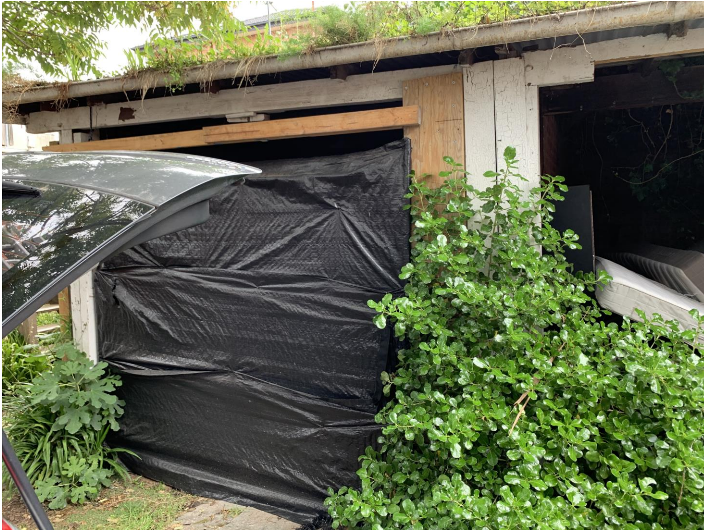
Image 9: Garages to the rear of the building. Source: M. Cooksley, 2020
