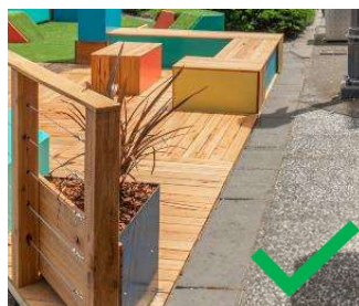
Figure 22: The platform has been constructed at the level of the footpath.
