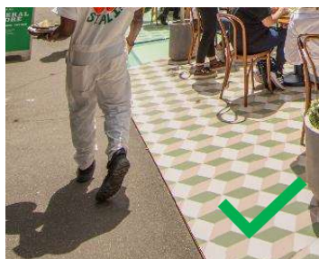
Figure 21: A mat creates a flush transition from the platform to the footpath
