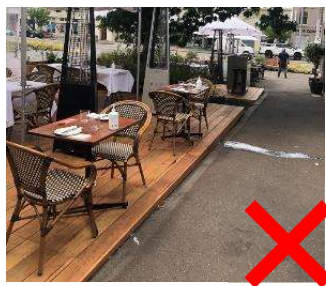
Figure 23: Platform is not flush with surround footpaths
