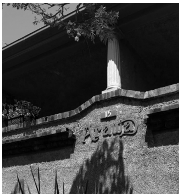
Photo 4. This block of flats in Wimbledon Avenue retains original finishes including the clinker brickwork, which contrasts with the natural (unpainted) render.
