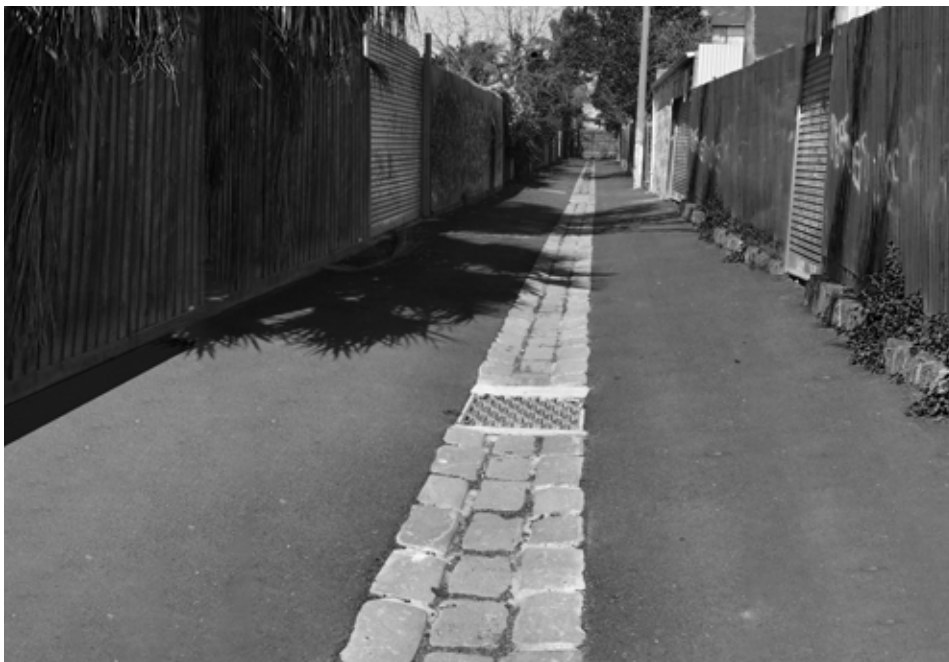
Photo 22. This laneway in St Kilda has been sympathetically re-constructed to retain the traditional bluestone channel and asphalt surface.
