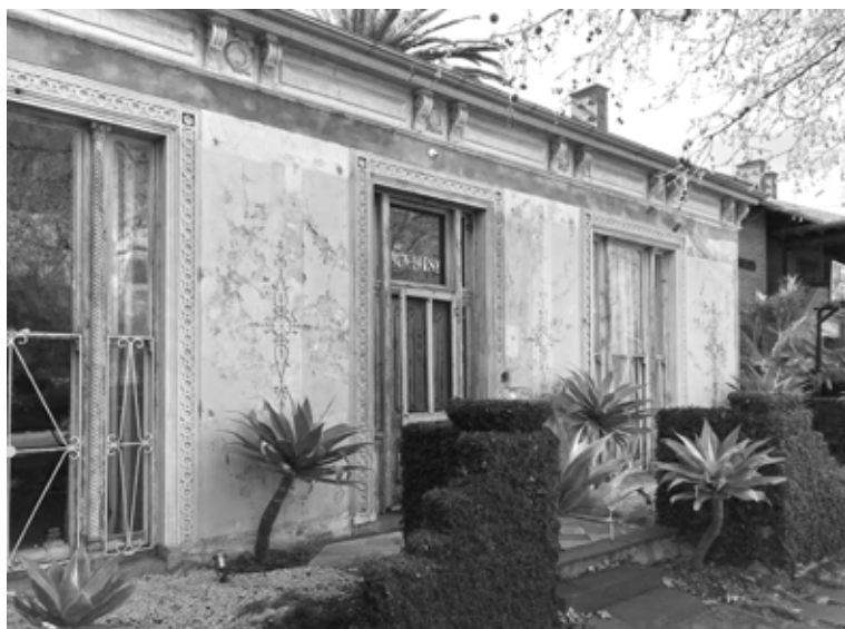
Photo 2. The removal of a c.1950s addition at the front of this house in Blessington Street, St Kilda revealed the original intact Victorian era façade. Outlines of the removed walls and some of the colour schemes, as well as the lower sections of the walls (now covered in vines) were left as evidence of this change.
