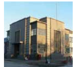
Former Chrysler building, 19 Salmon Street
