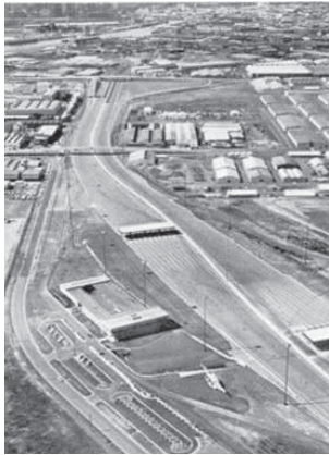
West Gate Freeway expansion
