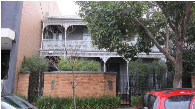
Figure 15 59-59a Wellington Street (Two-storey Victorian dwelling)
