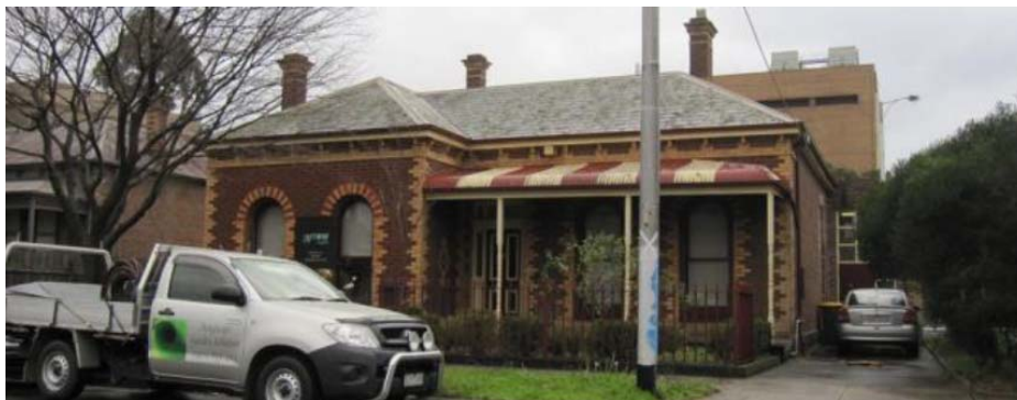
Figure 14 129 Wellington Street c.1885 single-storey bichrome brick Victorian dwelling
