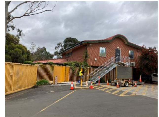
South Melbourne Operations Centre fire escape
