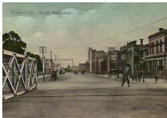
Figure 6.34-4 – Looking west along Bridport Street, c.1908
