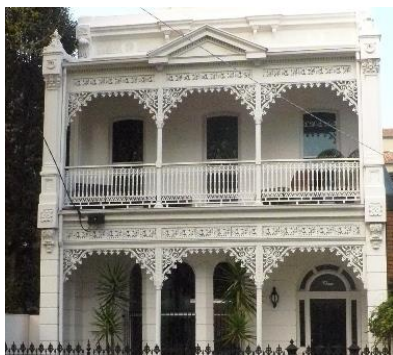
Figure 6.35-10 – Double-storey Victorian terrace house, Mary Street
