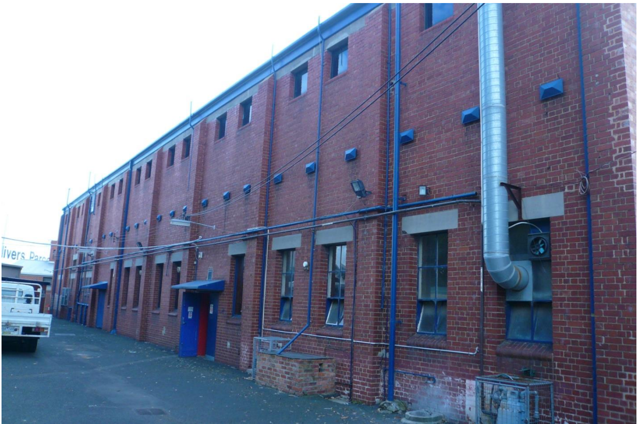
Figure 6.38-7 – Rear elevation showing unpainted brick and render finishes.
