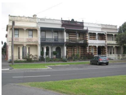
Figure 6.35-7 – Double-storey Boom-style Victorian terrace houses, Kerferd Road
