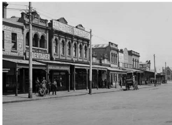
Figure 6.34-2 – Looking west along Dundas Place, c.1890s
