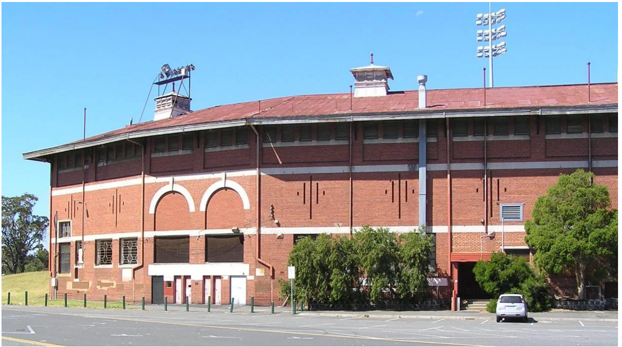
Figure 6.38–10 – The west elevation of the South Melbourne Grandstand, showing row of highlight windows beneath the eaves.
