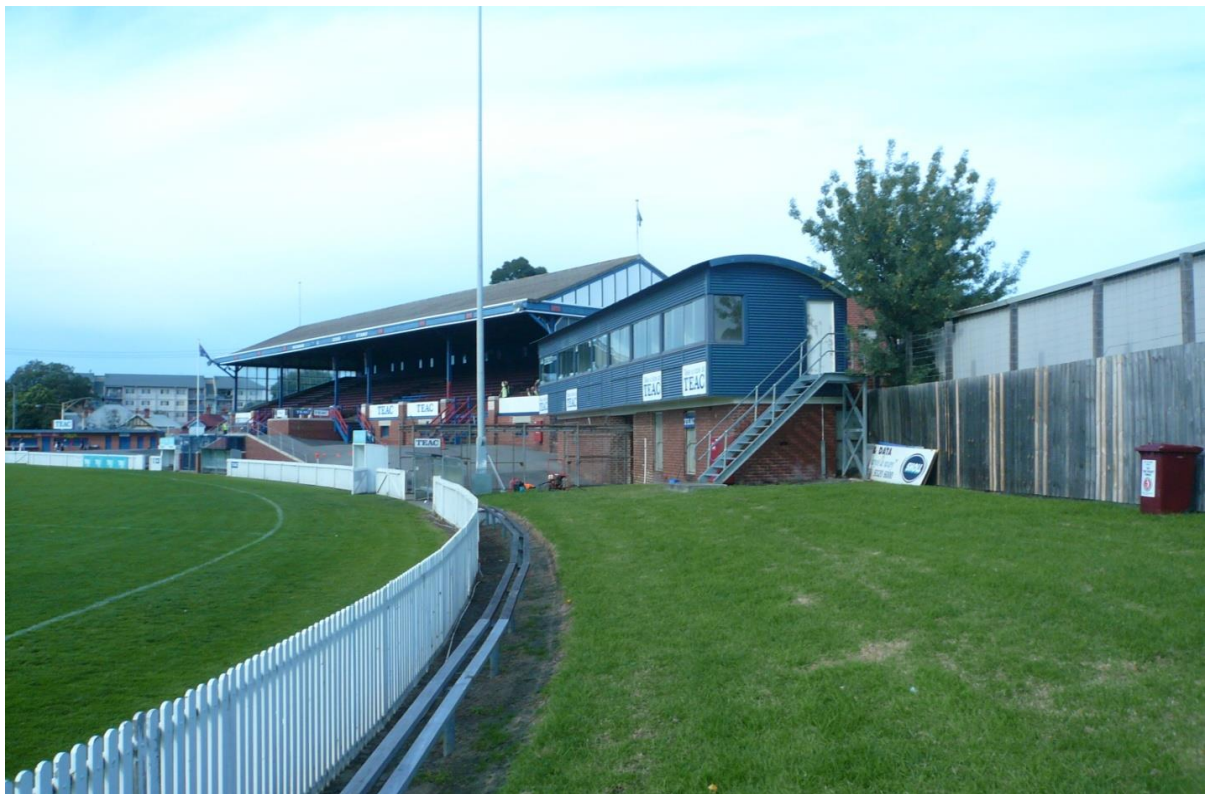
Figure 6.38-I – The ‘away’ team’s rooms with the 2001 addition in the foreground and the Norman L Goss Stand, looking east.
