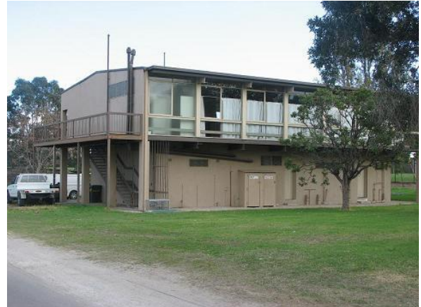
Figure 6.37-13 – One of the few surviving 1960s sporting pavilions, located near the John Blackham Oval
