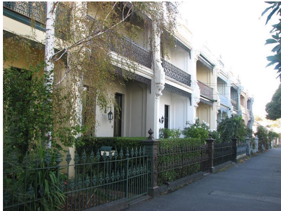
Figure 6.33–7 – A particularly fine row of double-storey rendered terrace houses in Montague Street
