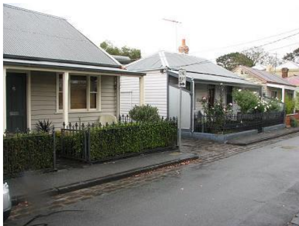
Figure 6.31-8 – Typical early double-fronted weatherboard cottages, in a row along south side of Thomson Street
