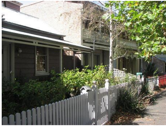
Figure 6.32-5 – Small single-storey timber villa at 16 Ferrars Place, and larger two-storey terraces at Nos 17-18.
