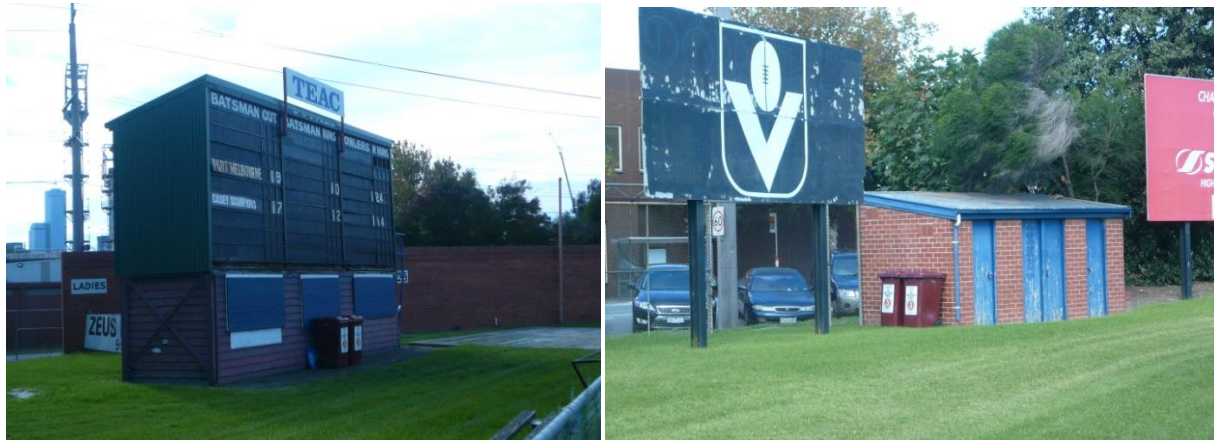
Figure 6.38–2 – From left: the scoreboard; hoardings and ticket entry kiosk to Ingles Street.
