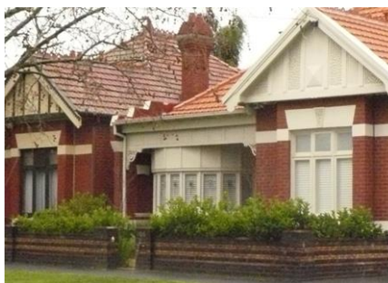
Figure 6.35-17 – Edwardian red brick villas, Nimmo Street
