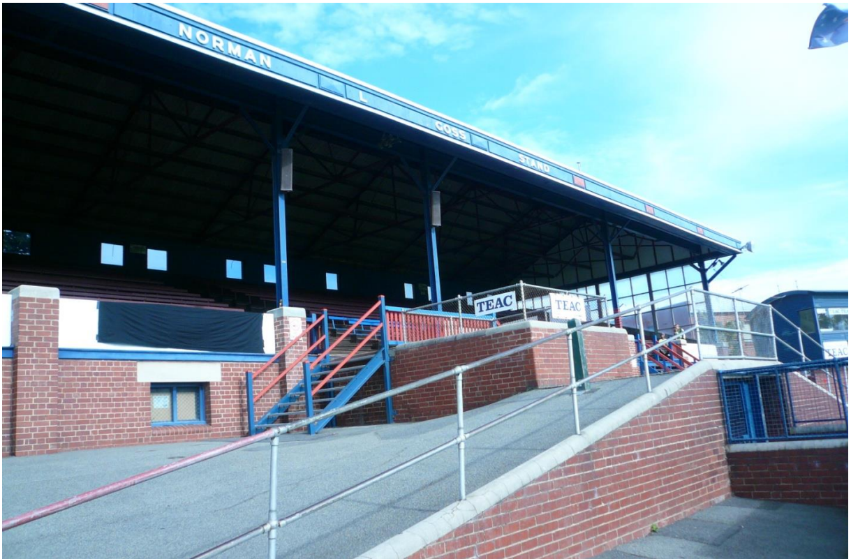
Figure 6.38-6 – Entry ramp and access stairs, Norman L Goss Stand.
