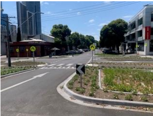
Raingarden and intersection improvements at Market and Clarke Streets South Melbourne
