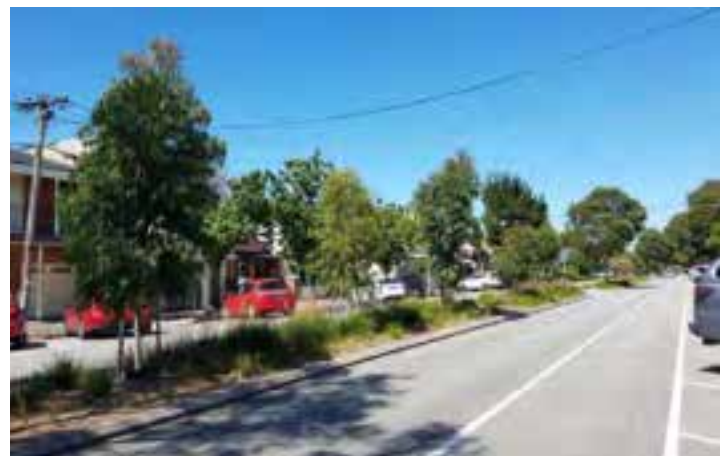
Figure 8: Recent work undertaken in in Bridge Street, Port Melbourne, provided an opportunity to depave the existing median, providing tree and understory planting opportunities to assist in mitigating urban heat island effect.
