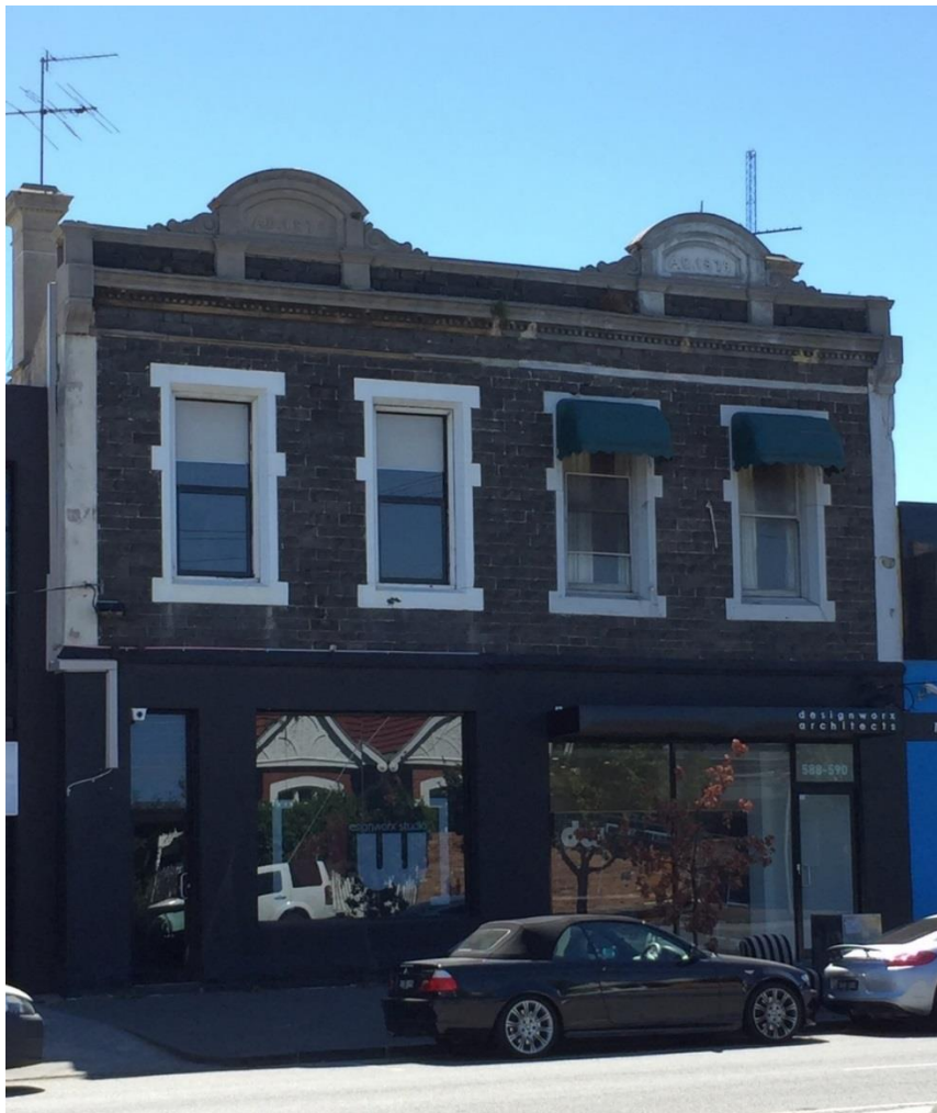
Figure 1. Image shows the pair of shops buildings with 588 to the right of the photo and 590 to the left. (Context 2017)
