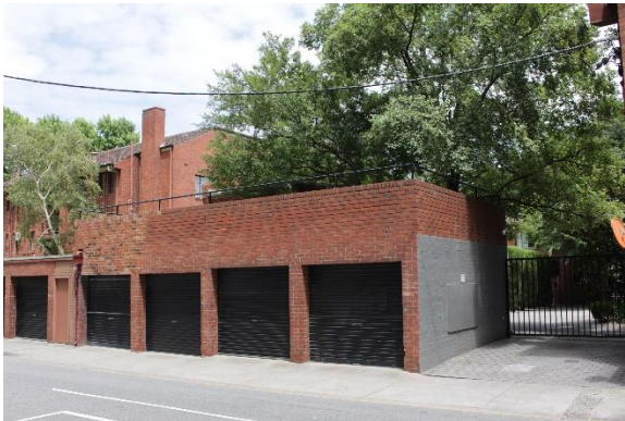
Queens Lane (rear) façade showing Glen Eagles (no. 58) to the right and original single car garages (x4) to the left, with outdoor clothes drying area above.
