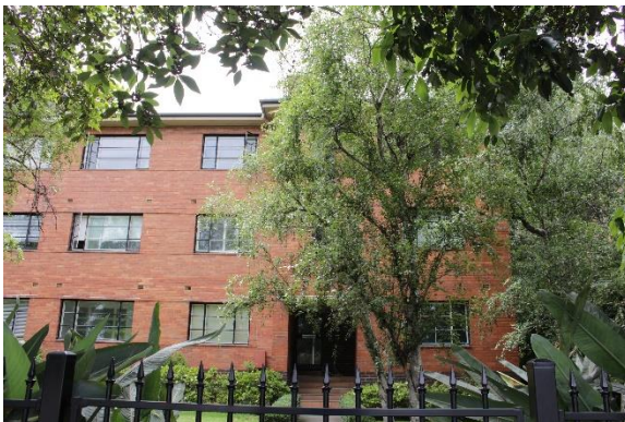
Glen Eagles (no. 58), Queens Road façade The projecting bay is just evident on the right
