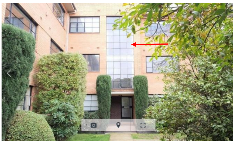
Kinross (no. 59), showing the west facing entry at the east end of the building. The projecting section is articulated by a large window of vertical proportions (arrow) and recessed entry with concrete canopy. (Source: onthehouse.com.au)
