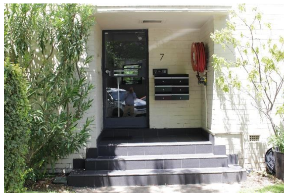
Monterey , showing recessed entry
