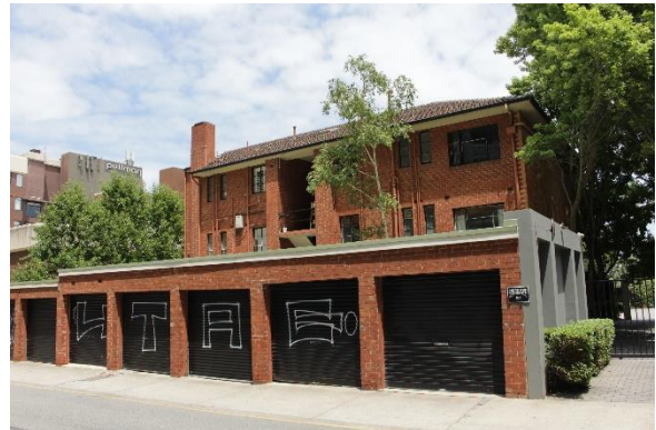
Queens Lane façade showing vehicular entry (right) between Kinross (no. 59) and Kinfauns (no. 60). The additional garages along the Queens Lane boundary had been constructed by 1945.
