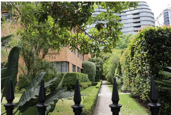
Kinross (no. 59), Queens Road façade from entry path and landscaping.
