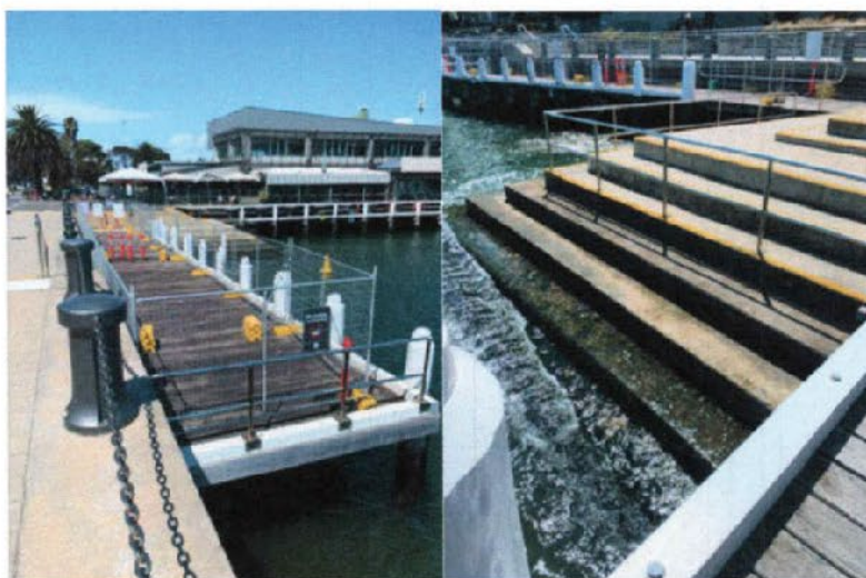
Lower Landing renovations
