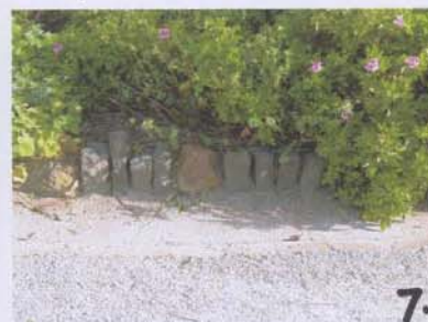
7. multiple rock types ok. (drystone edge)
