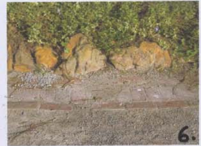
5. Good edge detail (local rock - sandstone spalls with brick channel) sympathetic to heritage
