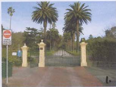
1. Main Entrance - Heritage gates missing gate → unbalanced symmetry
