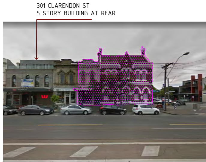
CLARENDON ST - FACING SUBJECT SITE
