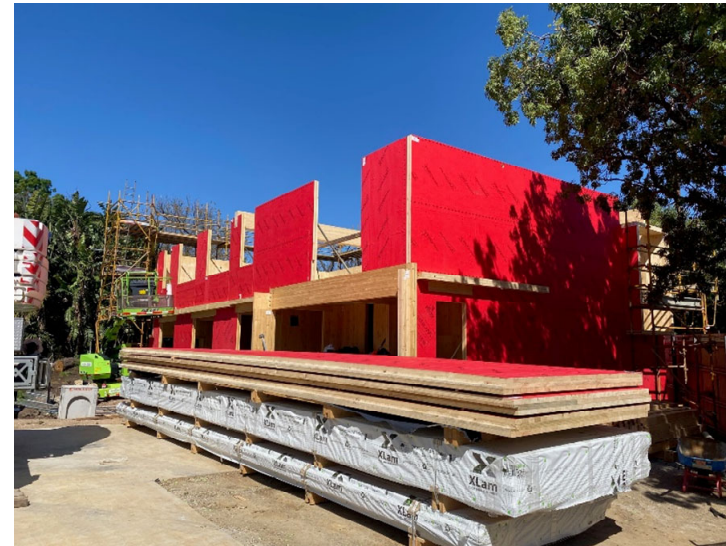
CLT framing being installed on the new EcoCentre building
