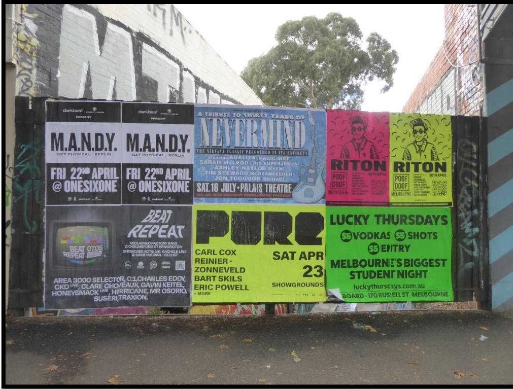
Eastern side – boundary of 362 St Kilda Rd. with the drain. Current timber paling fence w.5840 x h.2510mm.
