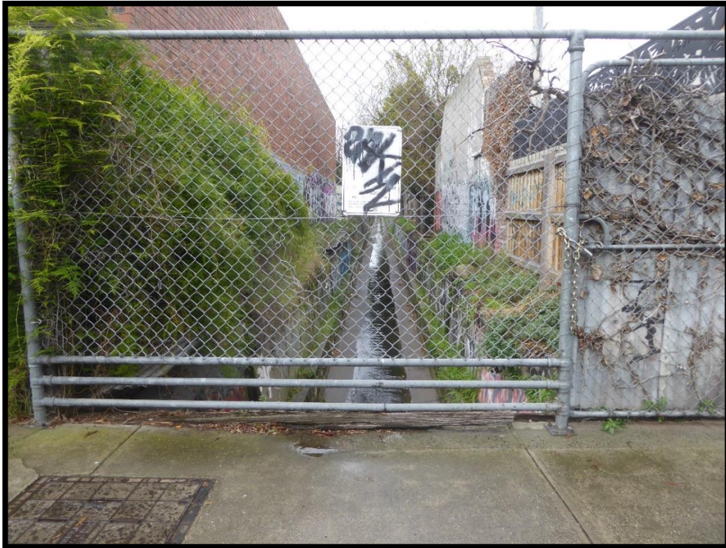
Greeves Street East cyclone fence barrier and gate W.4000 x H.2110mm.
