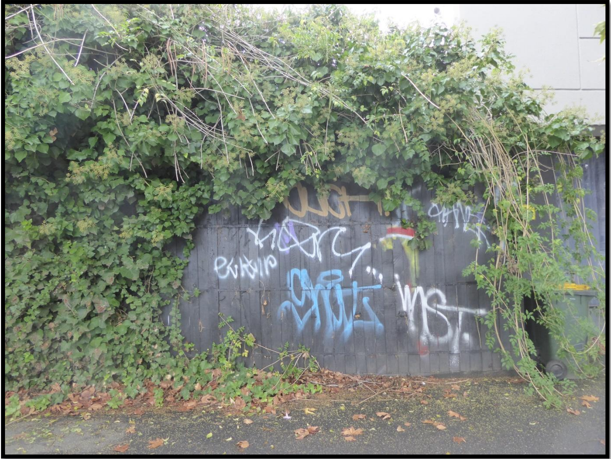
Western side – boundary of 345 St Kilda Rd. with the drain. Current timber paling fence w.4760 + corner return w.1200 x h.2470mm.
