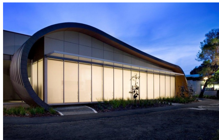
Betty Day Community Centre Architects: K20 Architecture
