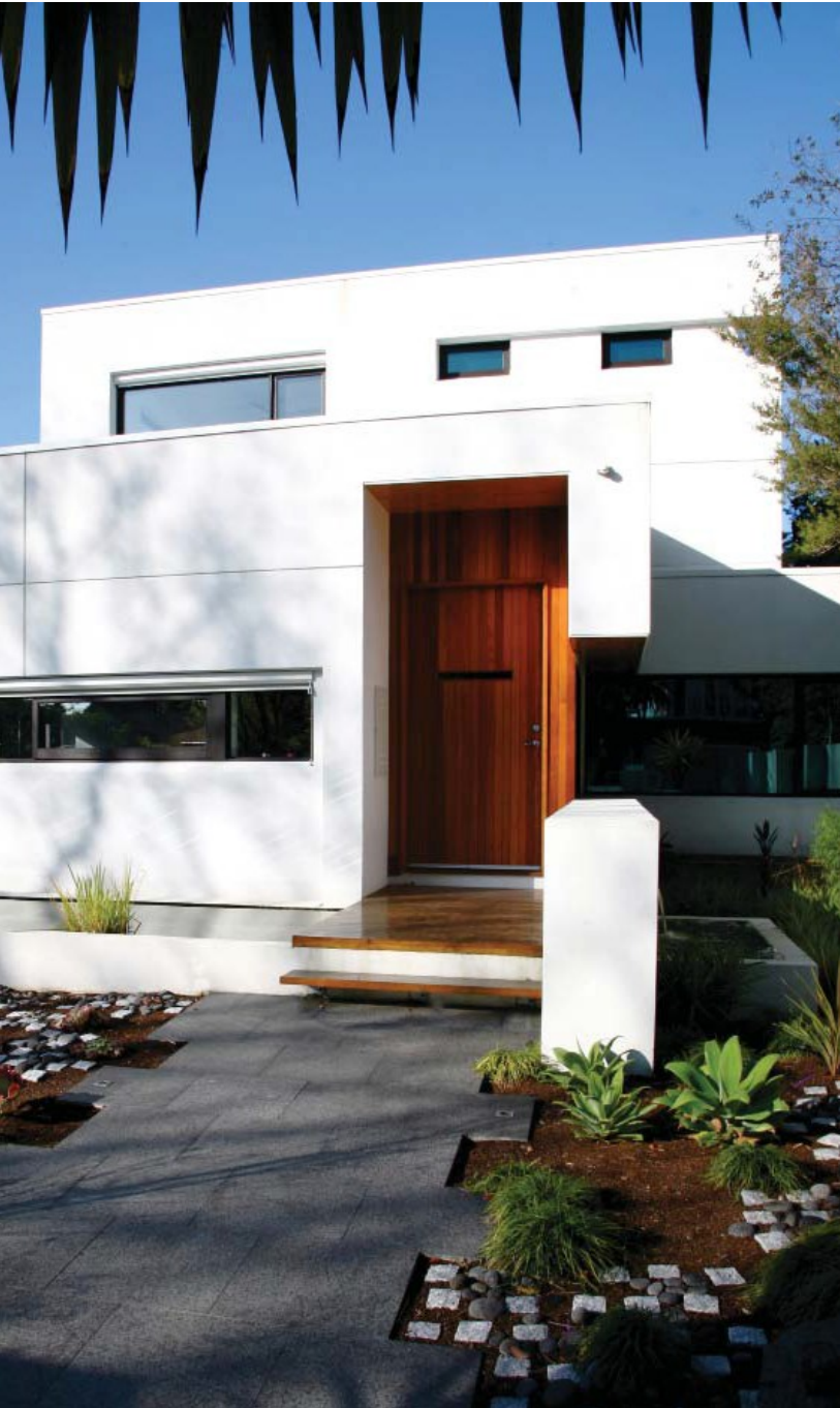
New Residence, Elwood.
