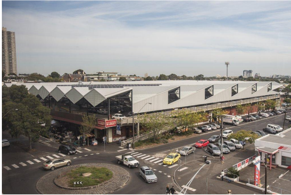
South Melbourne Market Roof Architects: Paul Morgan Features Include: 34kw Solar panels array and 500KL rainwater collection for re-use
